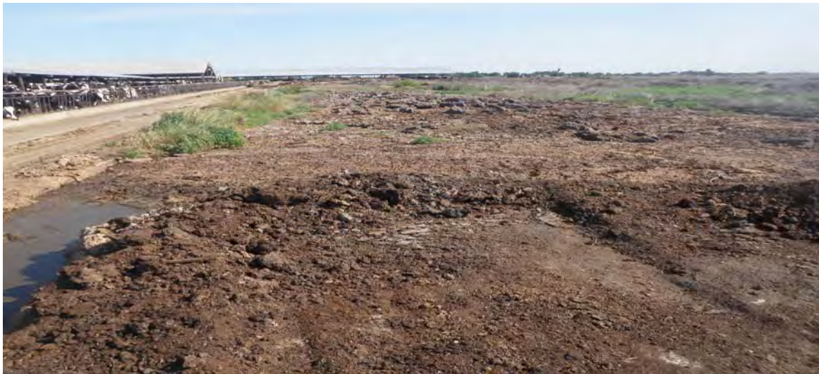
Photo 6: Looking north at the Settling Basin #1 (at capacity).
