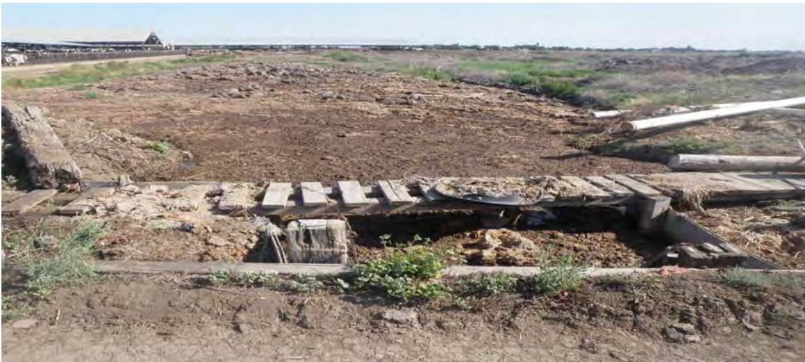
Photo 4: Looking north at Settling Basin #1.
