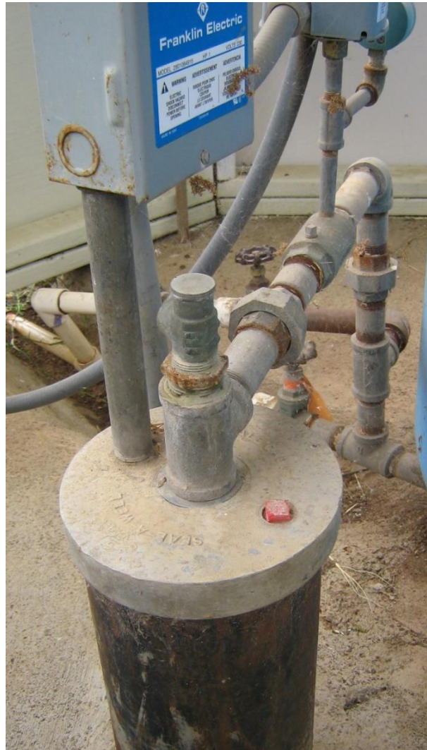
Figure 3. A typical domestic well head.
