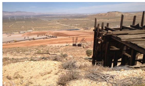
Figure 1: Heap leach pad being loaded with ore; black surface impoundment visible to the upper right of the heap; old mine works in foreground.
