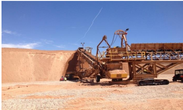
Figure 5: Cyanide solution conveyance piping. The black pipe conveys metal-bearing solution from the leach pad to the Plant, and the brown pipe conveys barren solution from the Plant back to the heap.
