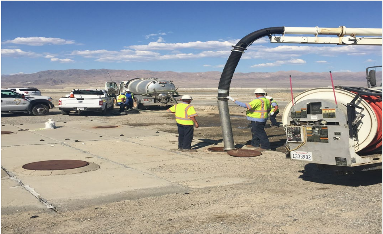
Figure 9.3 - View to east, main Trona septic tanks are pumped, cleaned, and inspected. Removed septage was disposed in the CSA 82 disposal ponds located on the east side of Searles Dry Lake.
