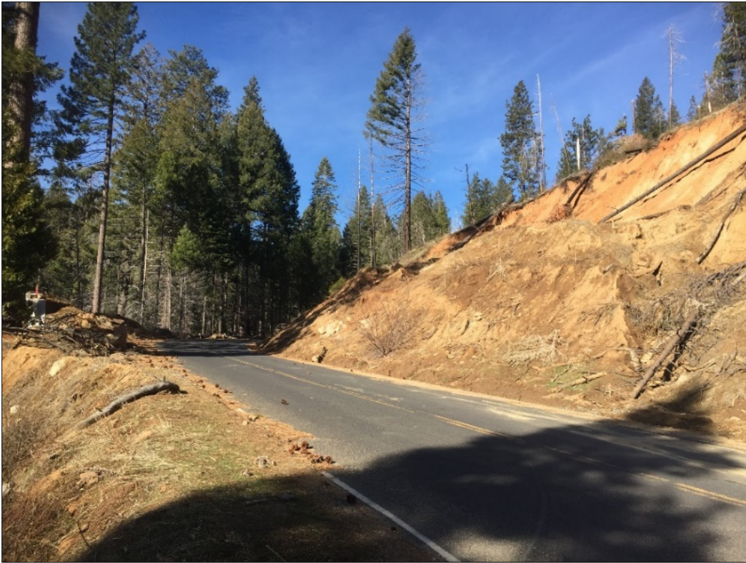
Figure 5.2 - Partially completed restoration of a landslide on a main timber access corridor. Hillside collapse occurred after a series of 2017 rain-on-snow events.
