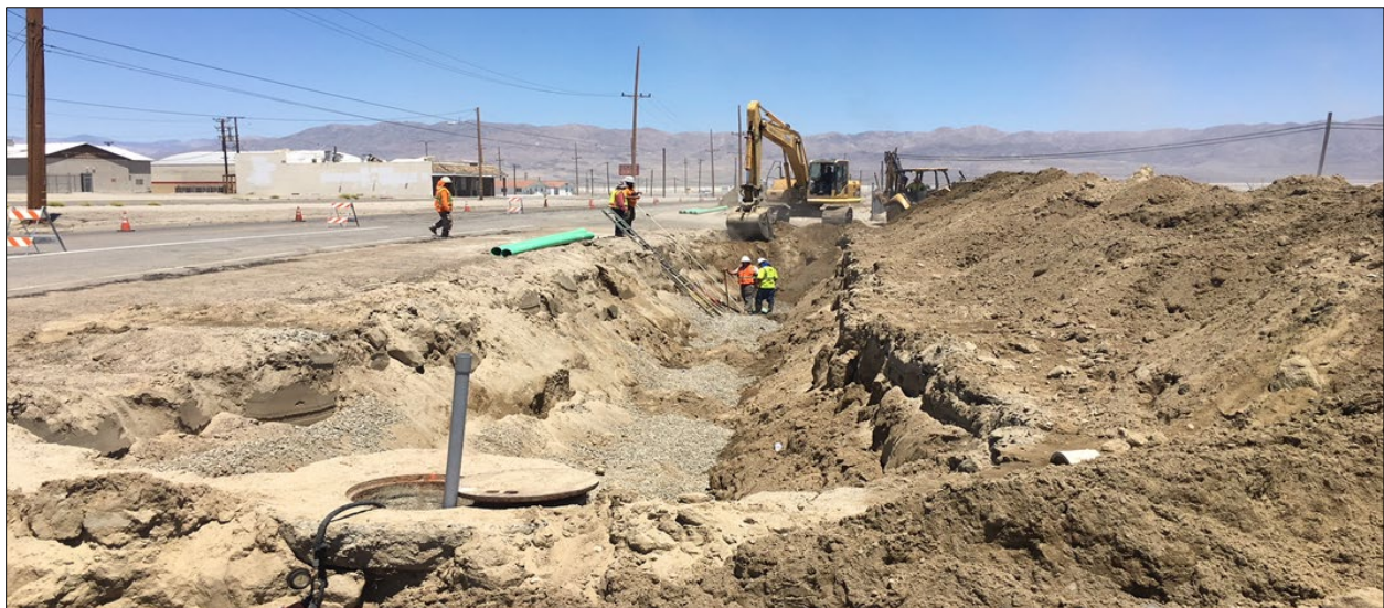
Figure 9.2 - View to north, along CA Highway 178, during replacement of failed collection system pipes.
