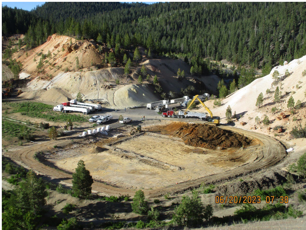
Photo 22 – June 20, 2023, Sludge haul activities at the Pit Clarifier.
