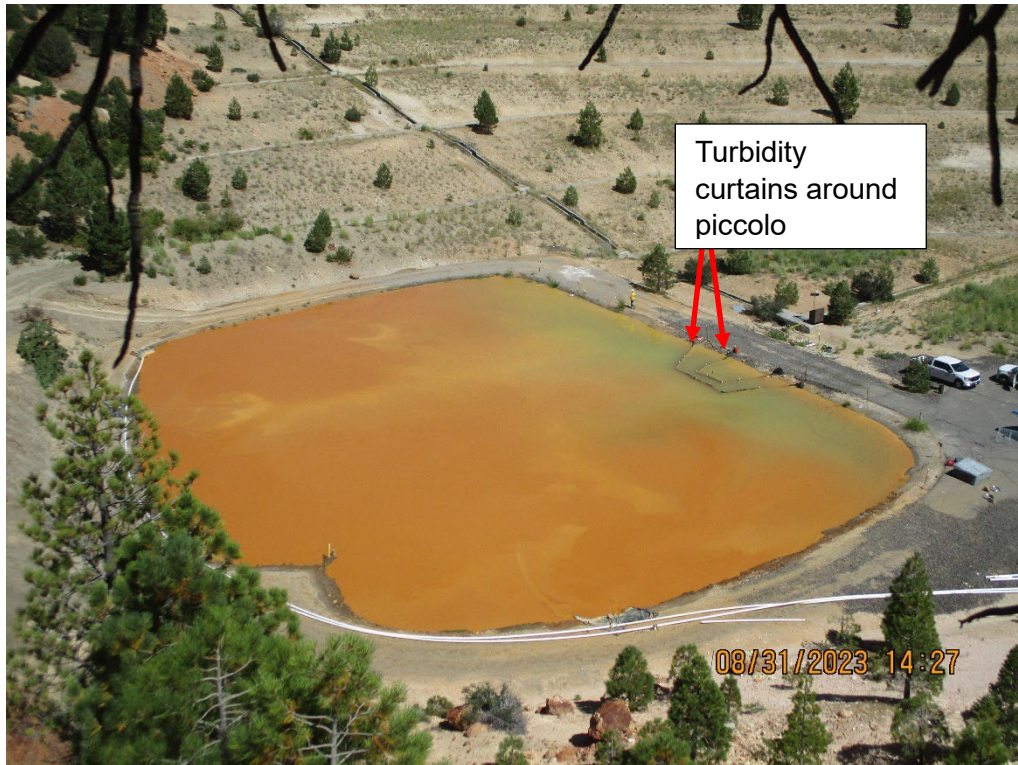
Photo 11 – August 31, 2023, Sludge buildup in the Pit Clarifier. Note the installation of two turbidity curtains around the piccolo structure.
