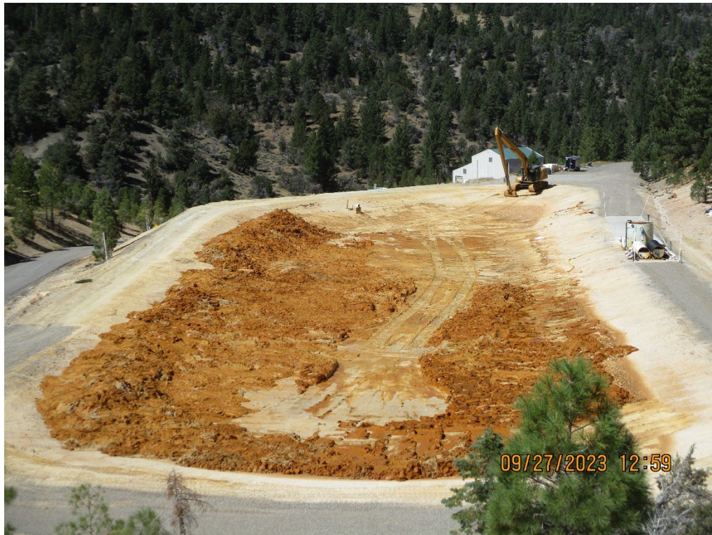
Photo 13 – September 27, 2023, Sludge stockpile activities at Pond 3. Much of the sludge was too wet to effectively stockpile at this time.
