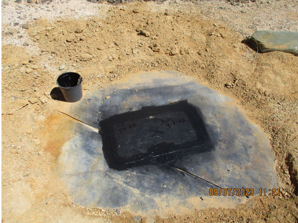
Photo 17 – September 7, 2023, Final Pond 1 liner patch on holes discovered in the fall of 2022.
