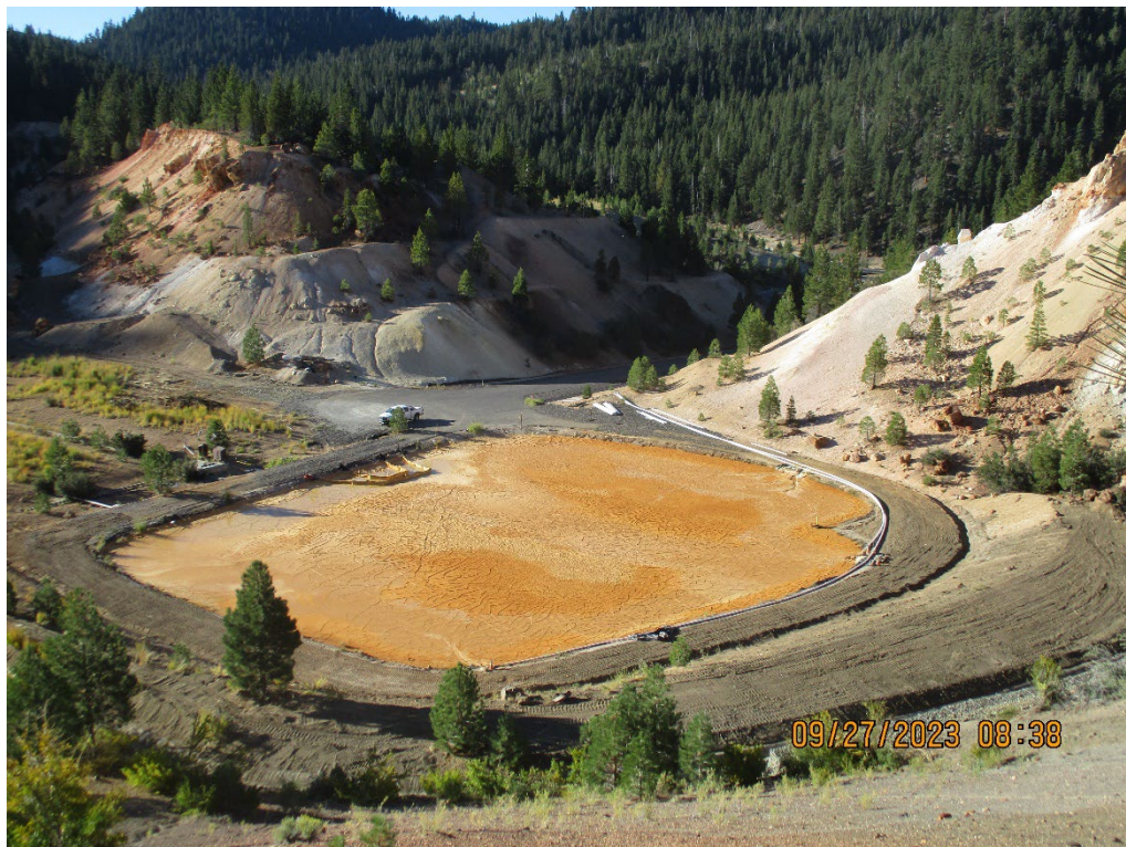
Photo 12 – September 27, 2023, The Pit Clarifier full of sludge shortly after Summer Pond Water Treatment was shut down for the 2023 season.
