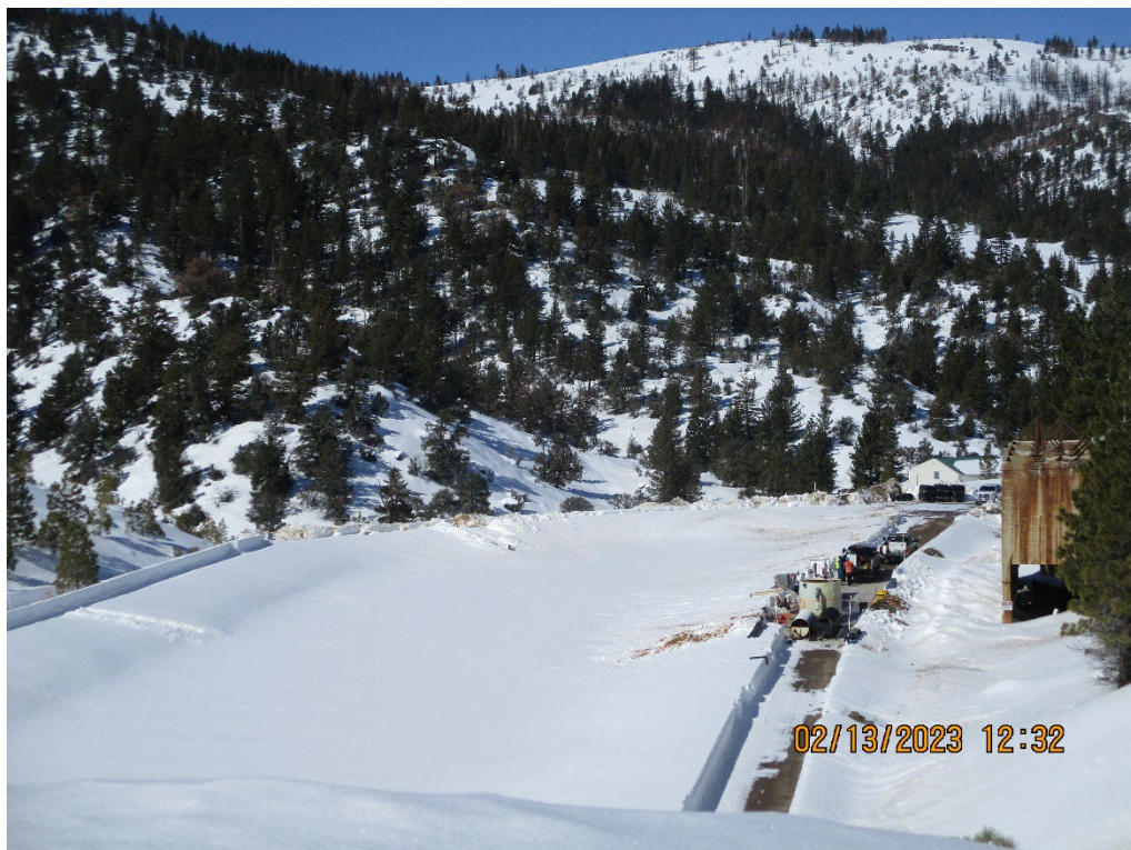
Photo 2 – February 13, 2023, TKT setting up Early-Season Pond Water Treatment system at Pond 3.
