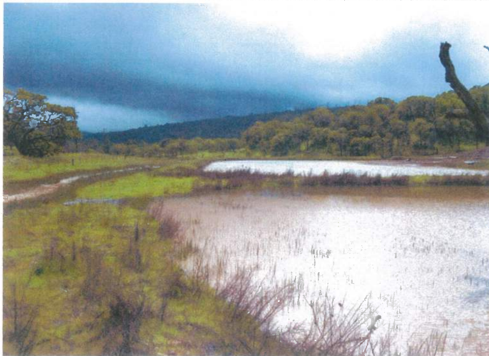
Photograph B-6: Storm water from upper mine working routed around the lower pond (right) via Dunn Creek (left).
