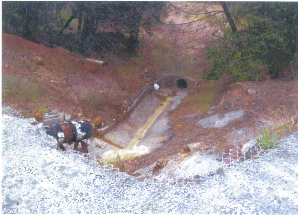
Photograph B-25: Surface water drainage from upper mine working area.
