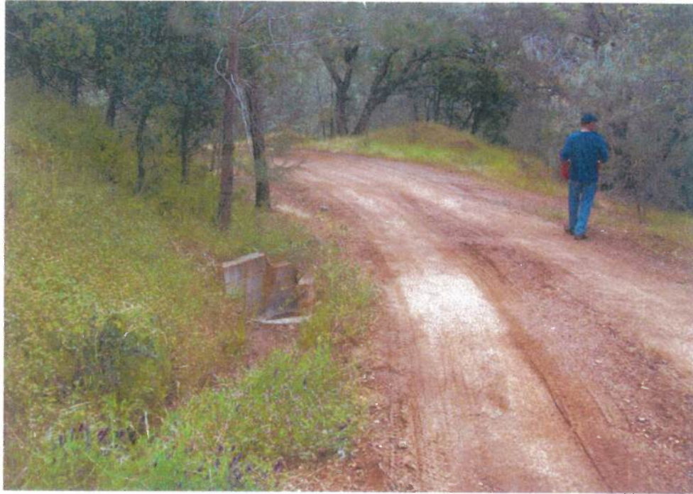
Photograph B-27: Drainage under road toward upper pond.
