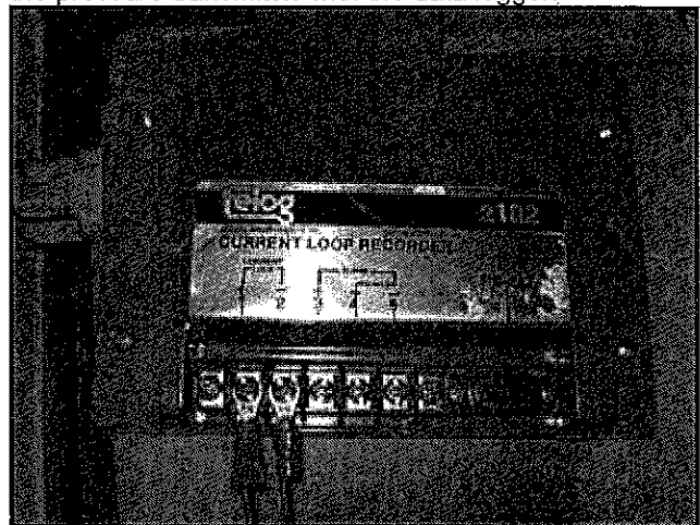
Photo 29. Telog data logger located near the transition from culvert to timbered section of the 700 Level Adit.
