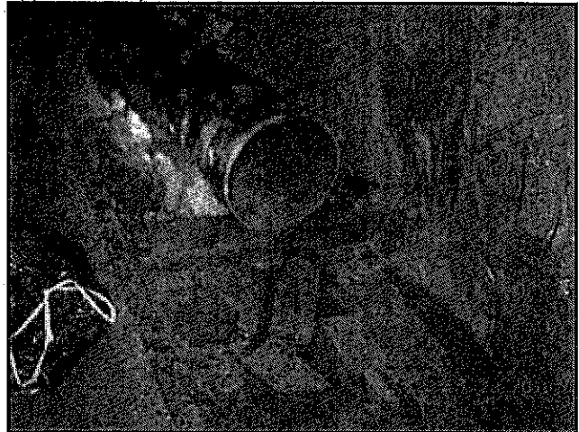
Photo 35. Showing termination of 18-inch ventilation ducting approximately 20 feet from the mine seal.
