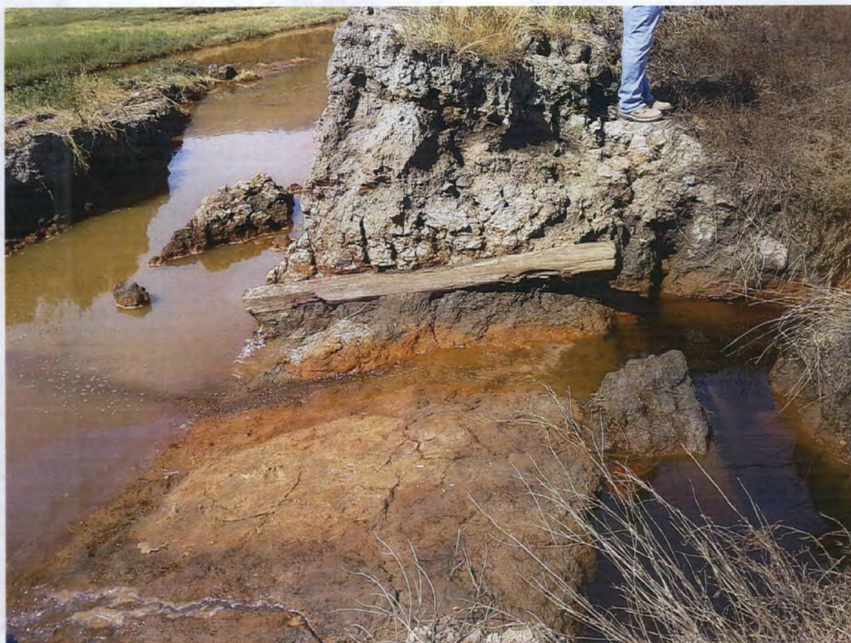
Photo 4: Breach 1 at First Levee Failure Location looking west at discolored water discharging from salt marsh into channel located on CDFW property.
