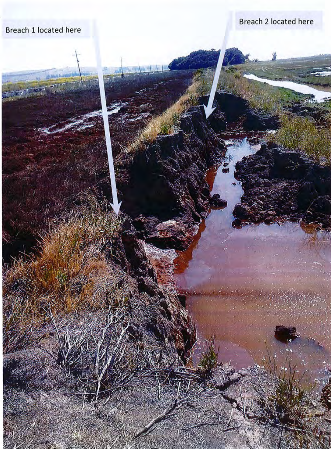
Photo 1: Two breaches at First Levee Failure Location looking east. Power lines to left are located on access road that separates the Mira Monte site owned by SMART from CDFW property, which includes the salt marsh to the left of the levee and the channel and seasonal wetlands to the right of the levee shown in the photo. The condition of the levee separating the two breaches is severely comprised and will likely fail if not addressed before it is exposed to high tides.
