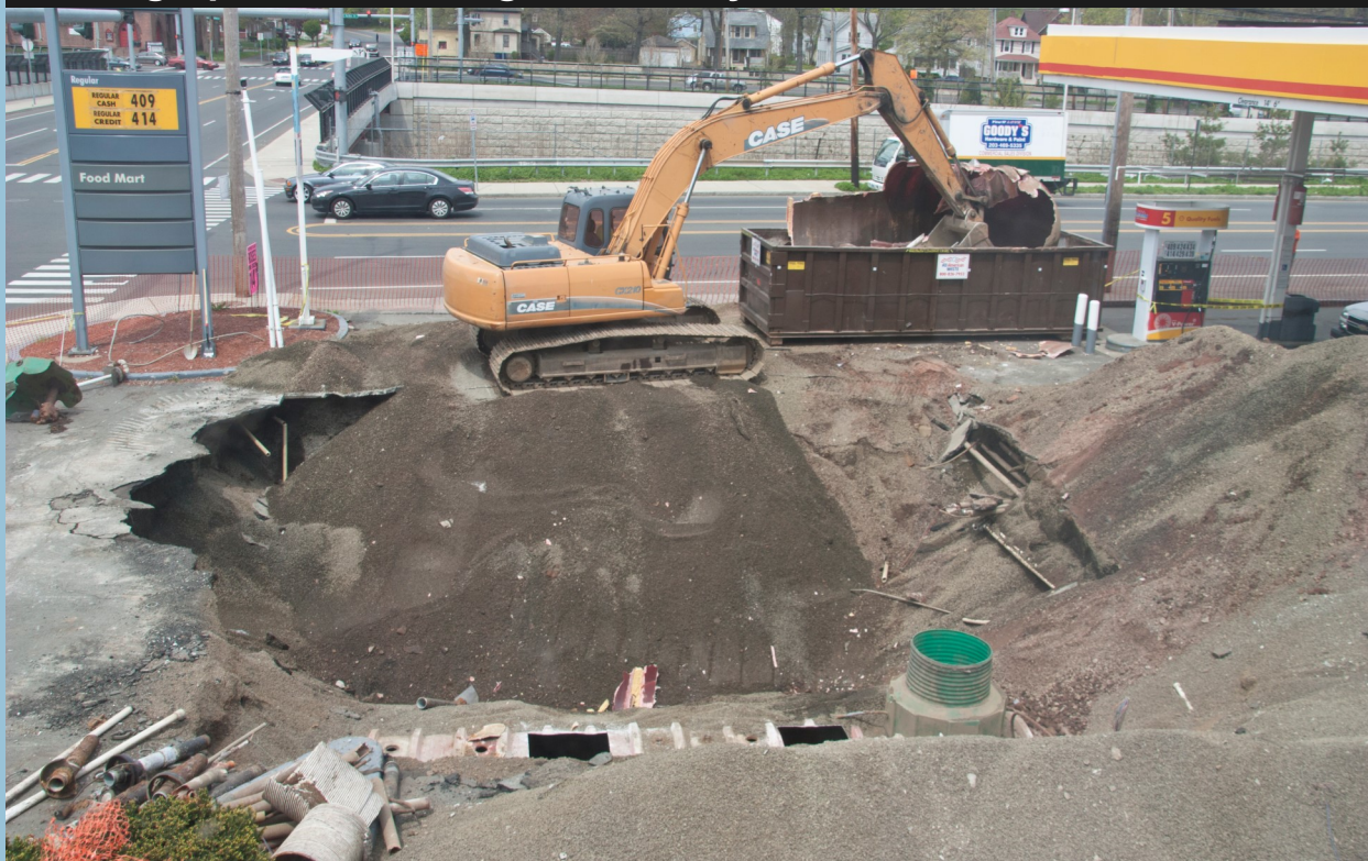
Photograph 1: UST being crushed by a backhoe
