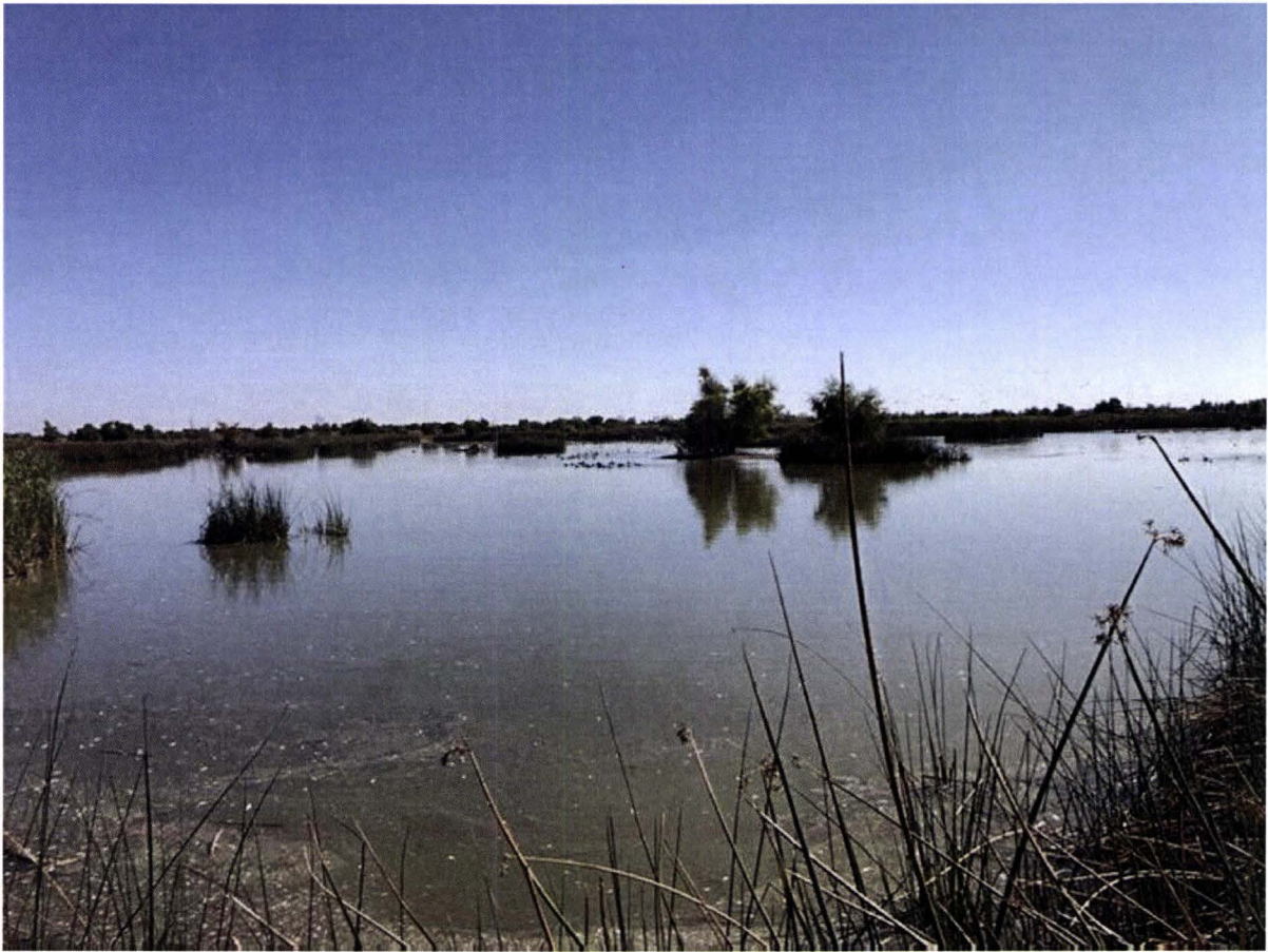
Figure 11: Wetlands Wastewater Track 10/5/22
