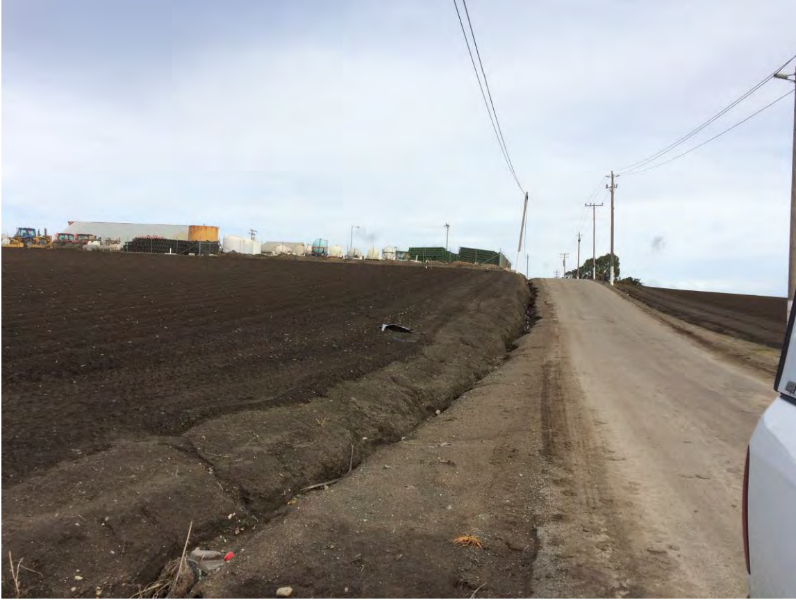
Figure 26. Photo of eroded road shoulder and channel along Boronda Road, west of the City of Salinas. Photo taken by staff on January 9, 2019.
