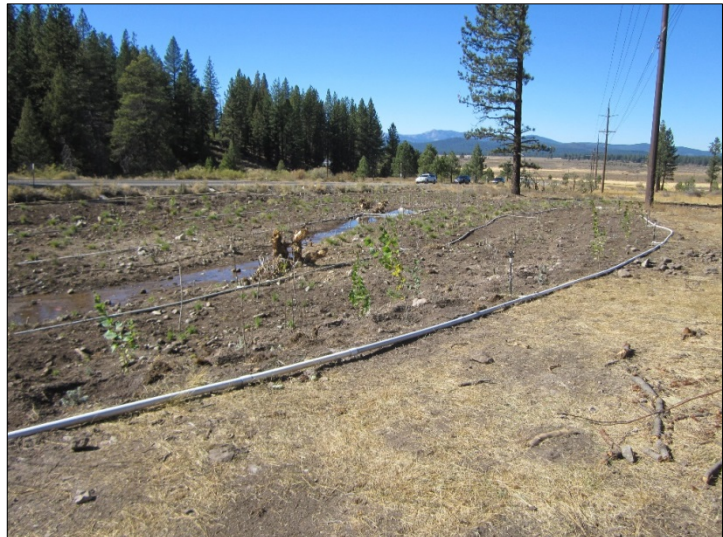
Photo 1: Restored creek bed, October 2016. (Photo courtesy of Truckee River Watershed Council)
