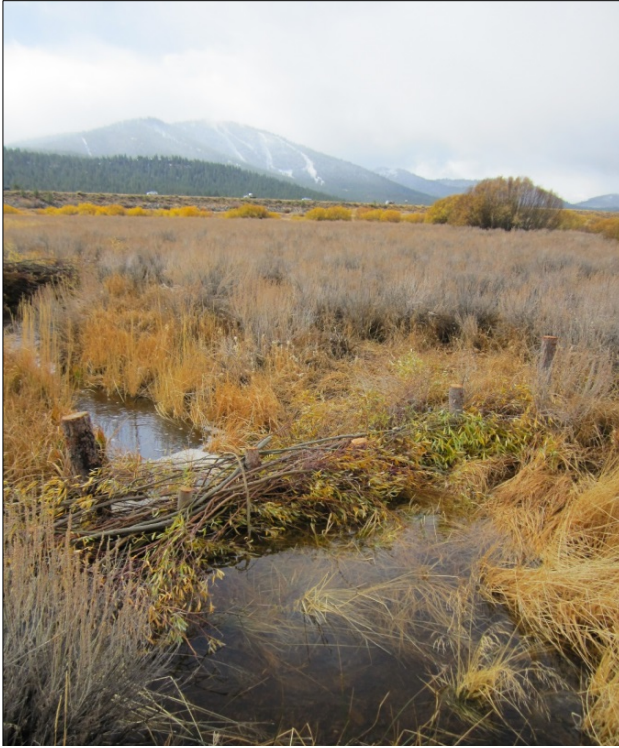
Photo 3: Functional Check dams after October 2016 storm event. (Photo courtesy of Truckee River Watershed Council)
