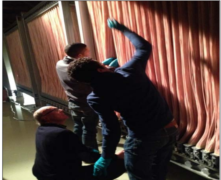
Photo showing a display of Membrane Bioreactor strands. These membranes are inserted into a treatment tank compartment.
