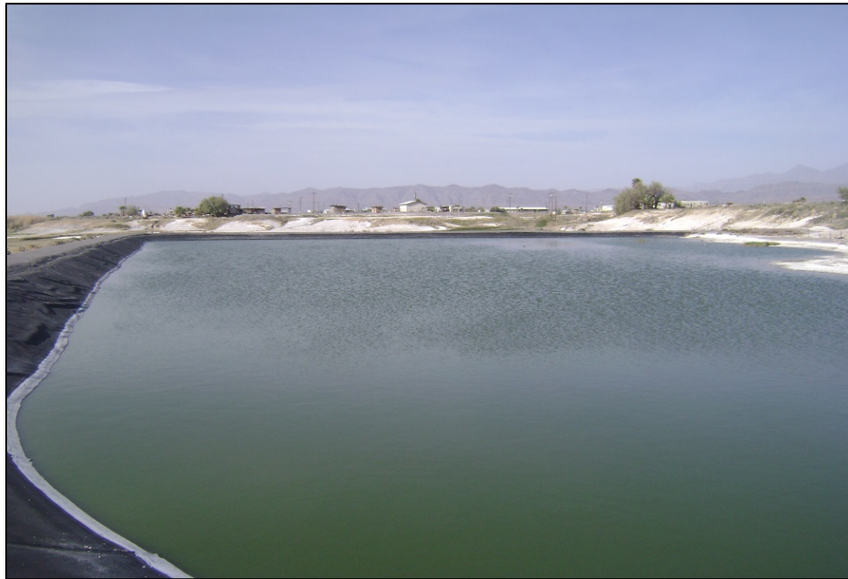
Photo showing the Inyo County Sewage Lagoon
