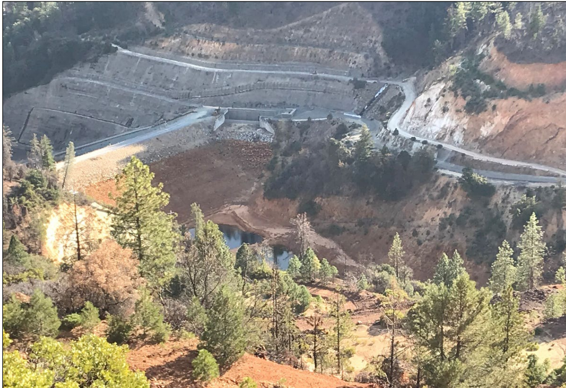
Figure 3.2 - Slickrock Creek Dam
