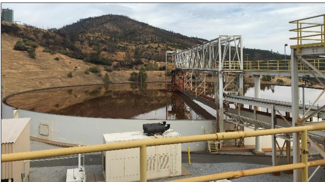
Figure 3.1 - Minnesota Flats Treatment Plant Clarifier
