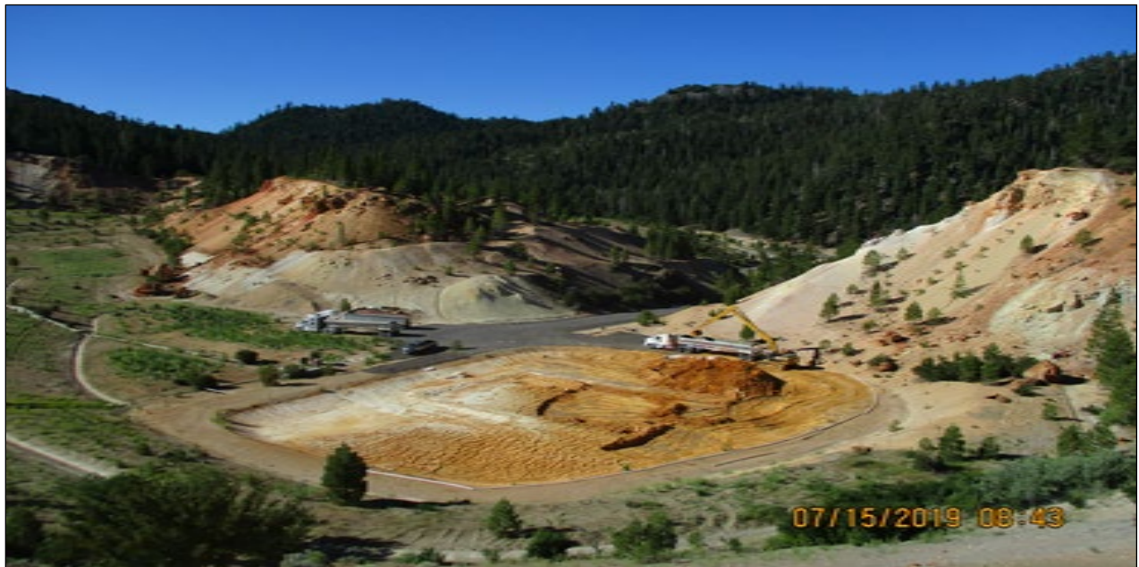
Figure 2.1 - Sludge Removal from the Pit Clarifier, July 2019
