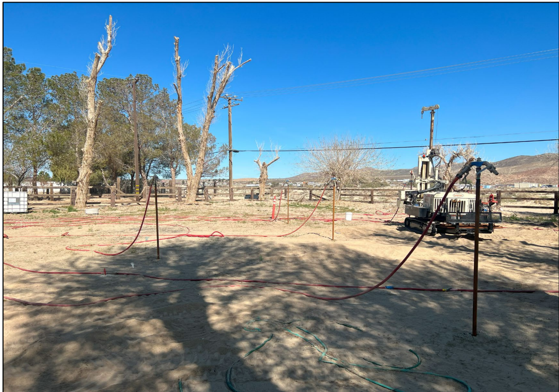
Photo 5.5: The “garden area” source zone, injection borings, and the direct push drill rig. Photo facing north.
