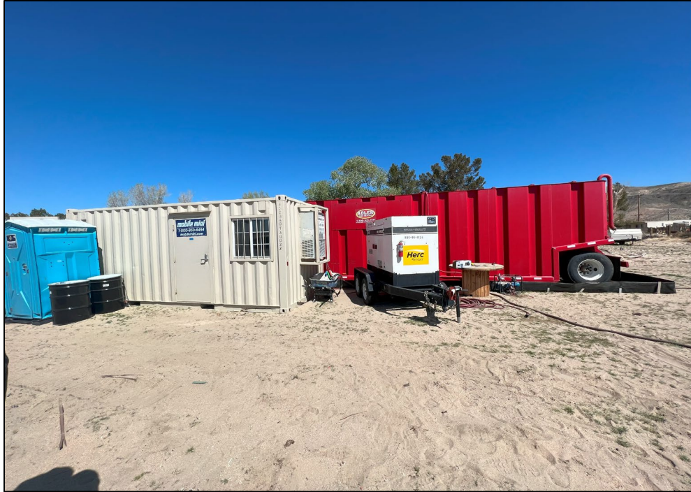
Photo 5.6: Water tank holding water used to mix with the EVO and mobile office for field operations located in roughly in the center of the treatment areas. The field office was also used to store field materials. Photo facing north.
