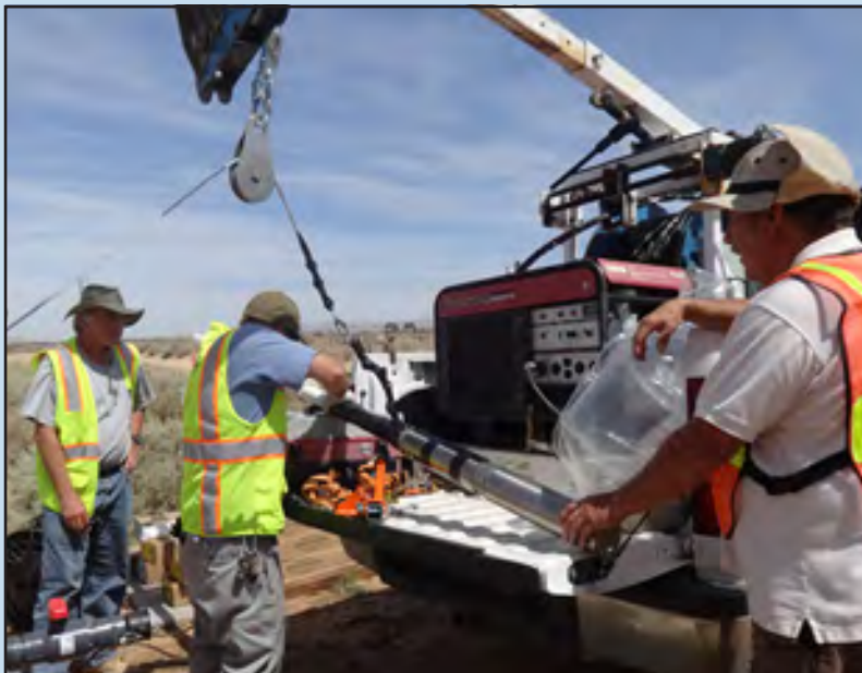
Figure 8. U.S. Geological Survey field crew preparing to set a temporary pump for borehole-geophysical data collection in a well, Hinkley, California, June 2015 (Roger Killian, Hinkley Technical Working Group, in foreground).
