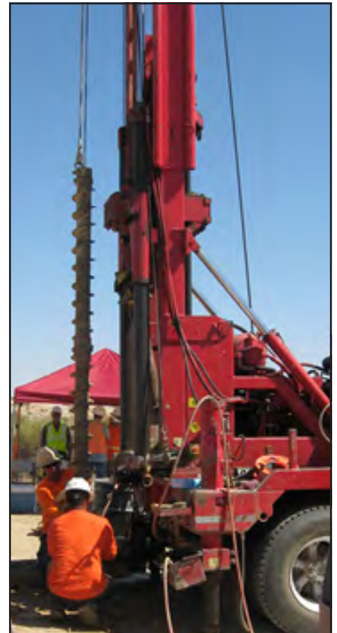
Figure 9. Test-drilling by consultants for Pacific Gas and Electric to install monitoring wells for flow-path studies, Hinkley, California, August 2015.
