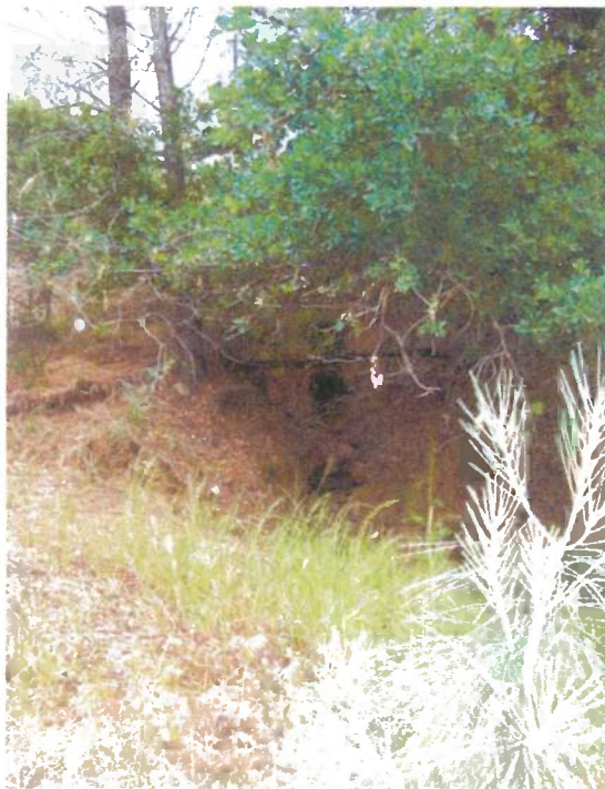
Photograph B-42: Surface water runoff channel to upper pond.
