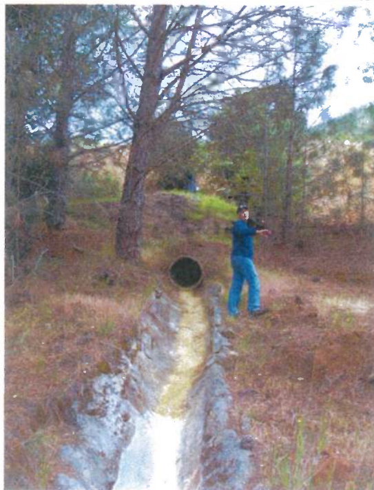
Photograph B-38: Storm water runoff outlet piping from upper mine workings area.
