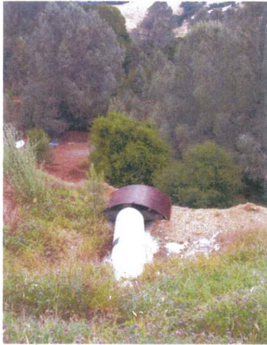
Photograph B-39: Storm water runoff outlet piping from upper mine workings area.
