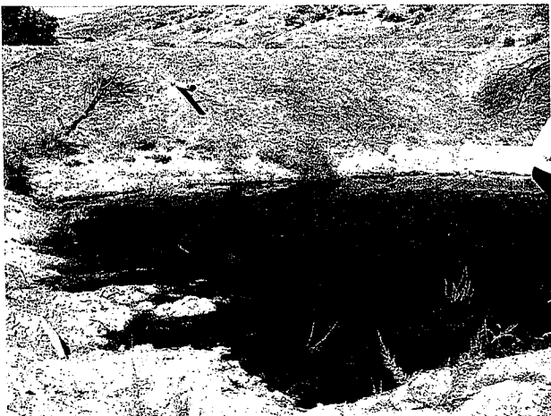
Photograph 5. – View of the elevated berm on Sump 26.
