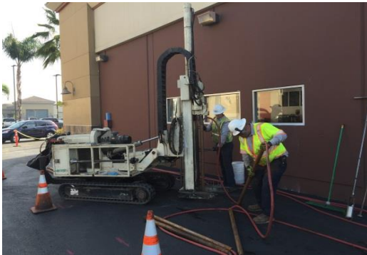
Advancing Injection Tooling
