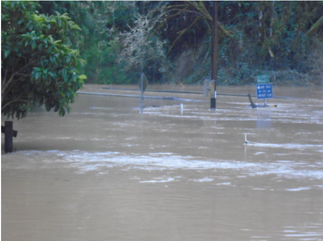
Figure 4: North Fork Bridge on Elk River Road at intersection with Wrigley Road. Note, only the guardrails of the bridge are visible. Photo taken by Kristi Wrigley on January 17, 2016.
