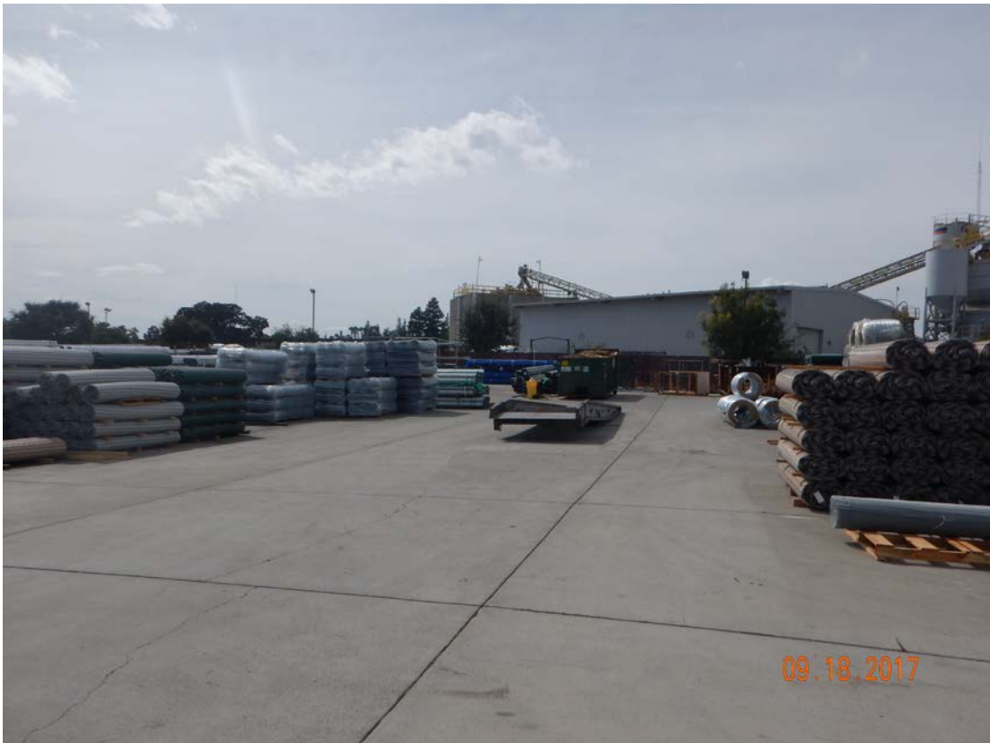
Photo 5. Another view of the southern portion of the Facility. The ground surface was clean and appeared to be swept regularly.
