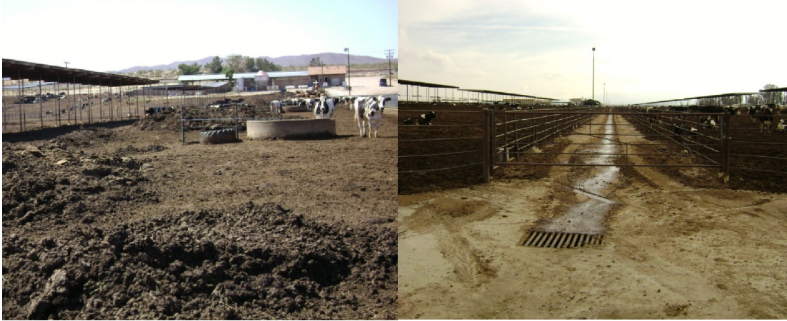
Neglected dairy corrals with excess manure piles and uneven ground. Photo by: Ghasem Pour-Ghasemi, Lahontan Regional Water Board.
