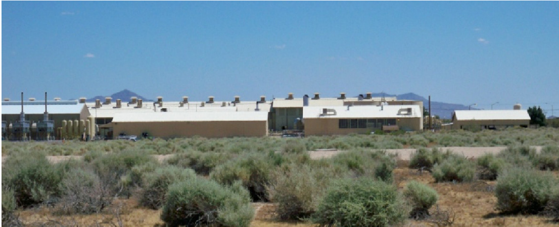
PG&E Compressor Station, Hinkley California. Photo by: Unknown.
