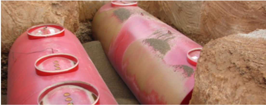
Underground storage tanks. Photo by: Amantha Henkel, State Water Board.
