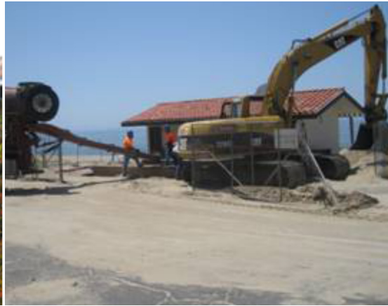
Point Dume Beach Restroom Under Construction. Photo by: Unknown.
