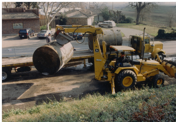
Tank Removal. Photo by: Unknown.
