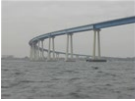
San Diego Bay Bridge
