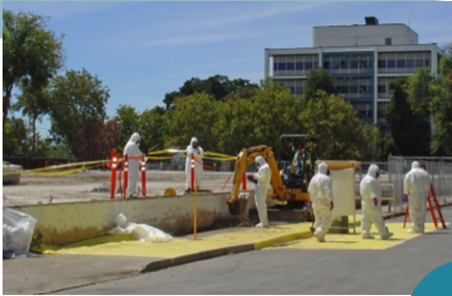
Photo to right: Removal of mercury from soil at Lawrence Livermore National Laboratory, a DoE site
