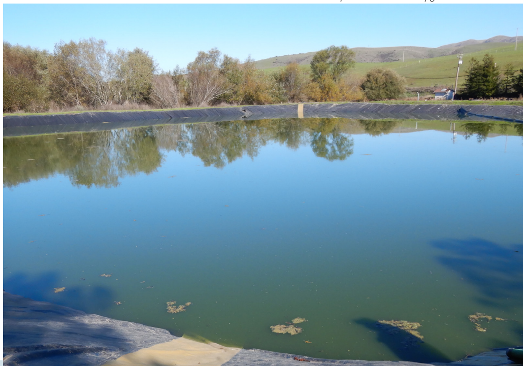
Photo below: Wastewater pond at Olema campground
