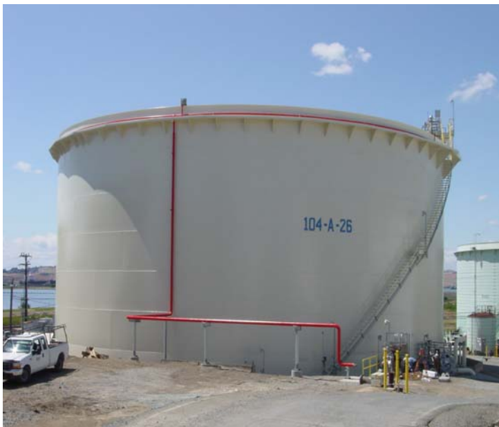
Photo 2: New Double Bottom Tank with Leak Detection
