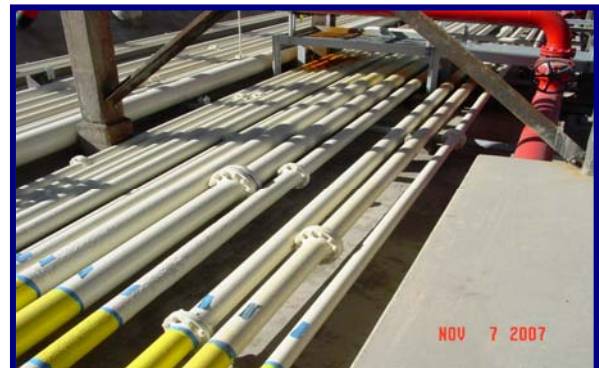
Photo 4: Upgraded pipelines –After
