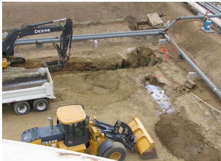
Installation of the interception trench in Gasoline Release Area
