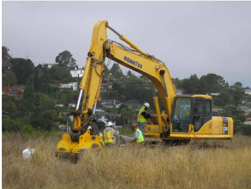
Heavy equipment moving on to Aramburu island
