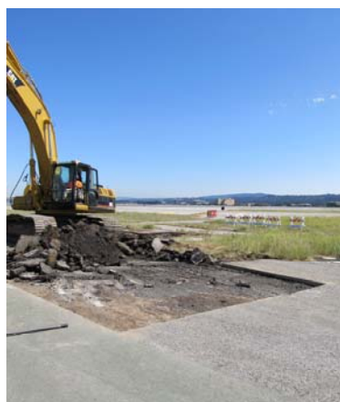
Photo 1. Excavated Taxiway Paving
