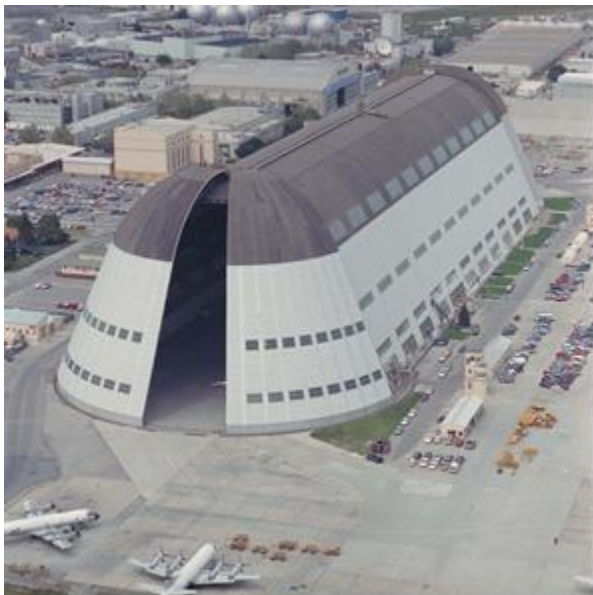
Photo 2a. Hangar 1 before siding removal.
