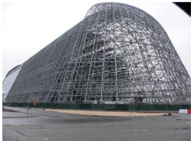
Photo 2b. Hangar 1 with more than half the siding removed.
