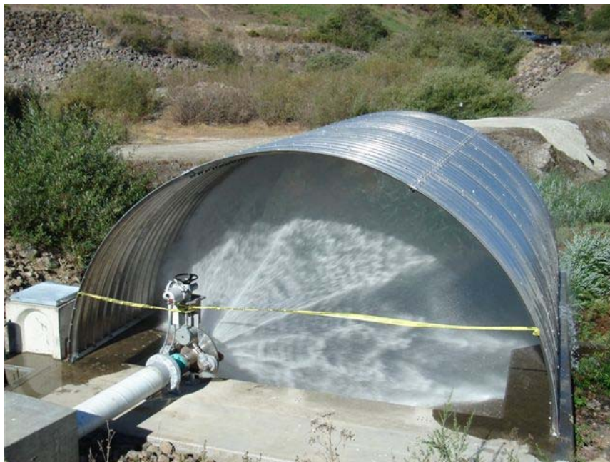
Photo 3. Valve installation with steel cover preventing bank erosion.
