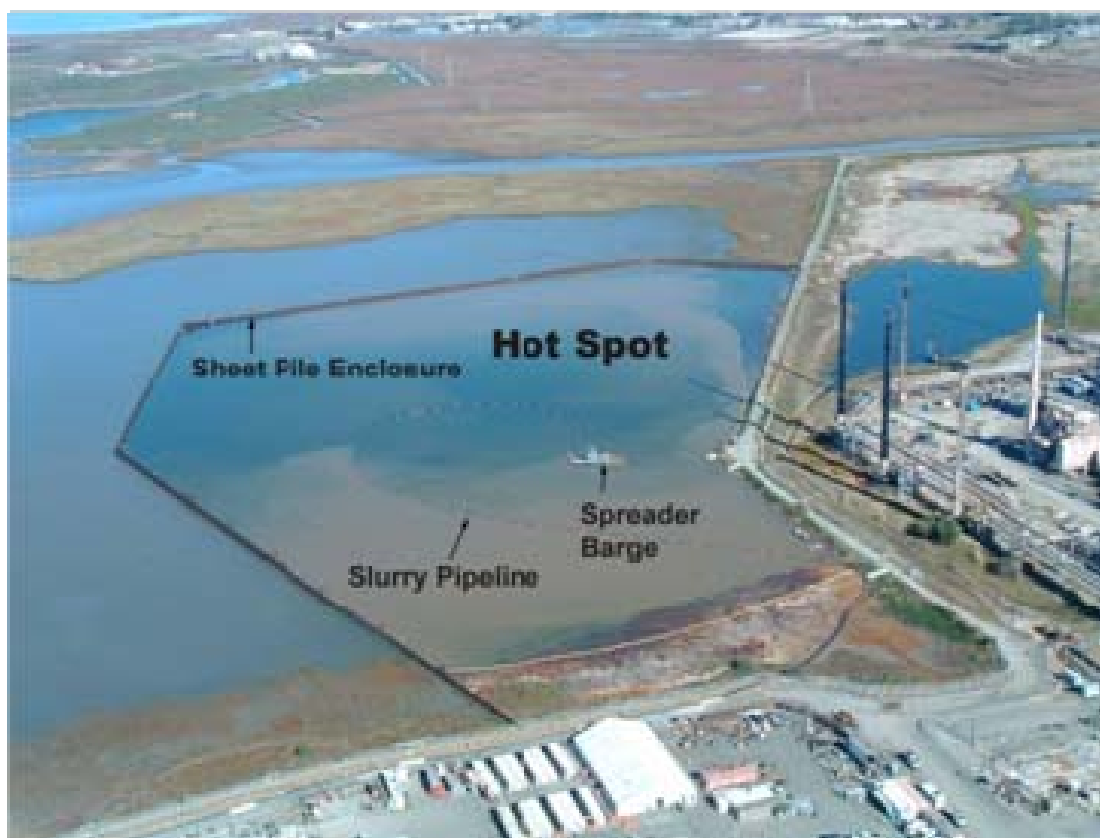
Image 2b. Castro Cove Remediation, November 2010
