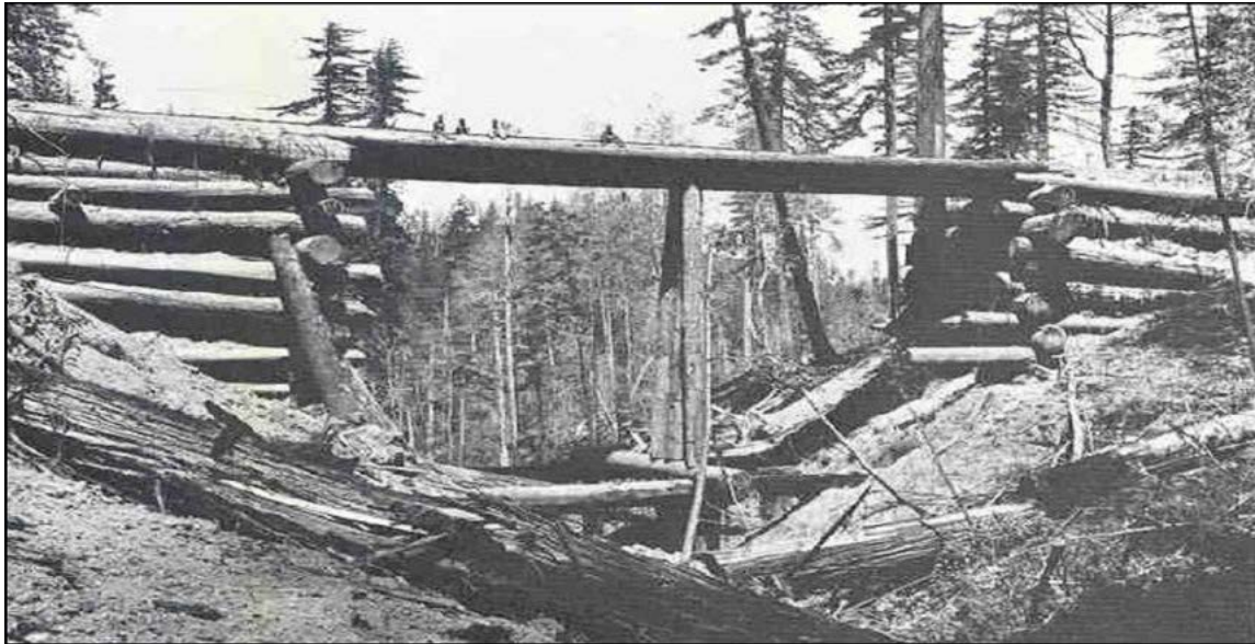
Figure 1. 1940s photo of Dark Gulch crossing construction
