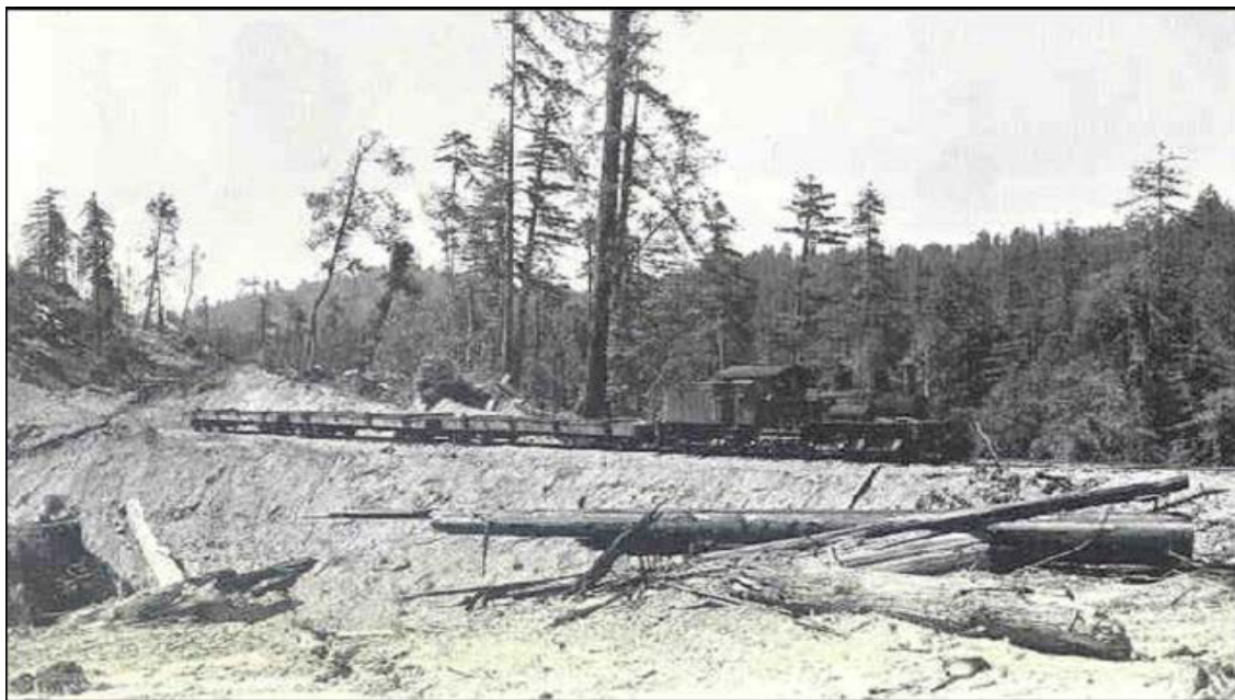
Figure 2. Example Humboldt crossing in Santa Cruz Mountains
