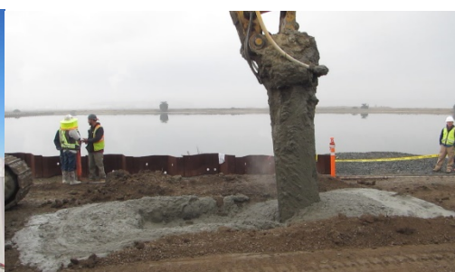
Injection of Grout Slurry
