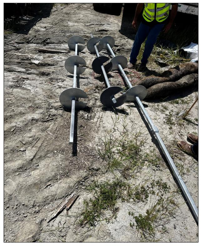
Figure 3. Guy anchors for the net poles that hold the barrier netting, waiting to be dropped into an open boring. Tensioned wires run from the corner net poles to these anchors.
