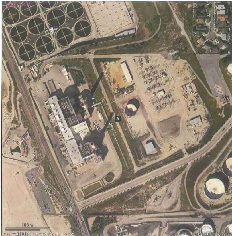
Figure ES-5 - Aerial view of Scattergood Generating Station
