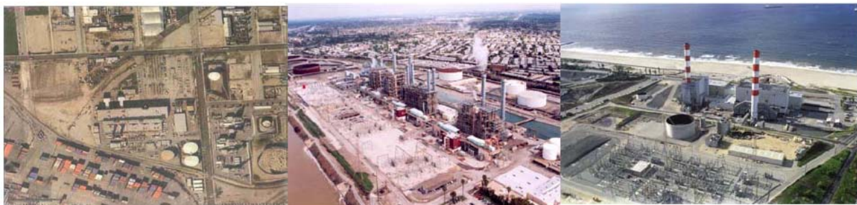
Figures 1 – 3 – Harbor, Haynes and Scattergood Generating Stations – Aerial photos
