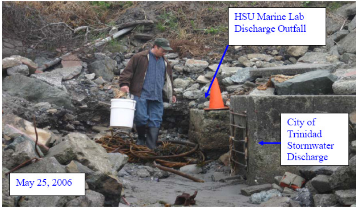
Photo 7.1.7.2. Discharge Points: Seawater System Outfall SCCWRP ID# TRI 033
