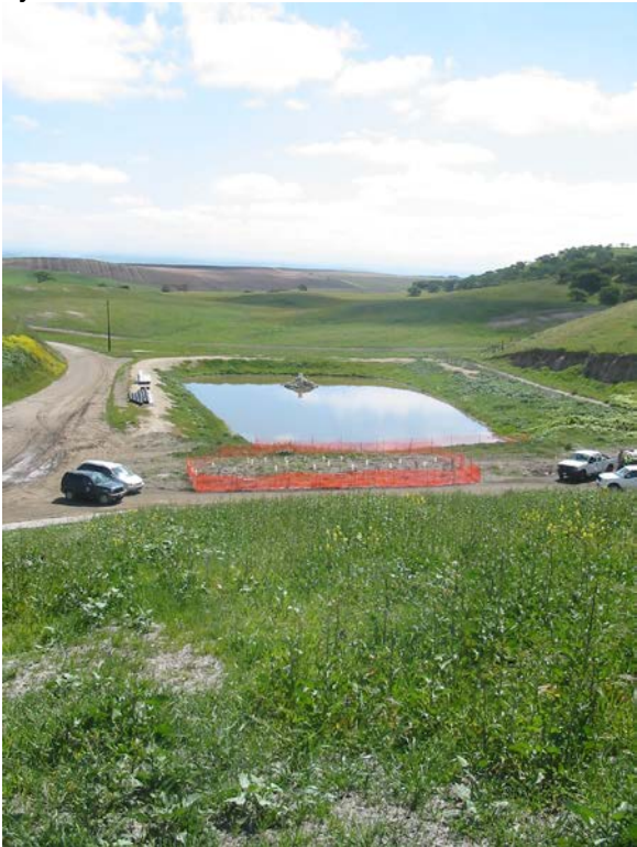
Photo looking east taken during final cover inspection at Jolon Rd. Landfill in January 2008. Healthy cover growth in foreground, and view of phytoremediation pilot study plot between the sediment retention basin and top deck.
