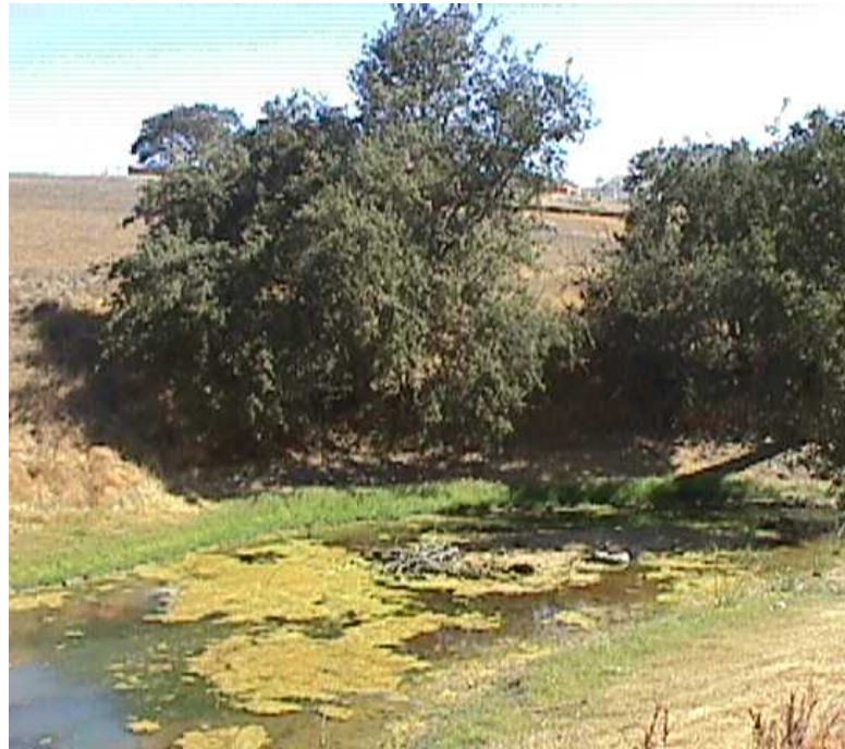
October 2002 – Pond in natural drainage was filling in from erosion caused by drainage overflow and sediment from construction site upstream. Pond and riparian area (not shown) contained construction debris, which demonstrated the source of the sediment and fill material.
