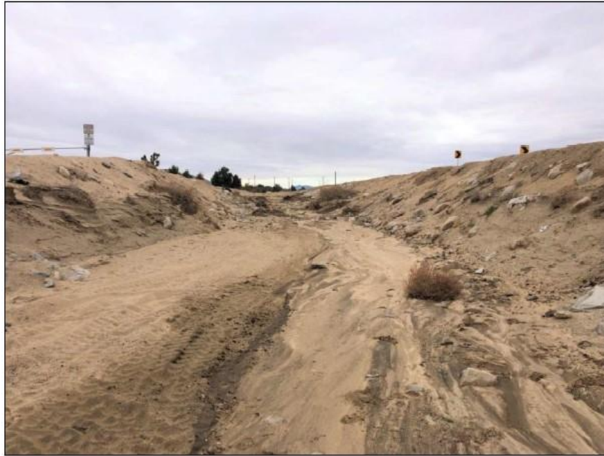
Figure 7. Photograph of impacted area PM 0.3, westside.
