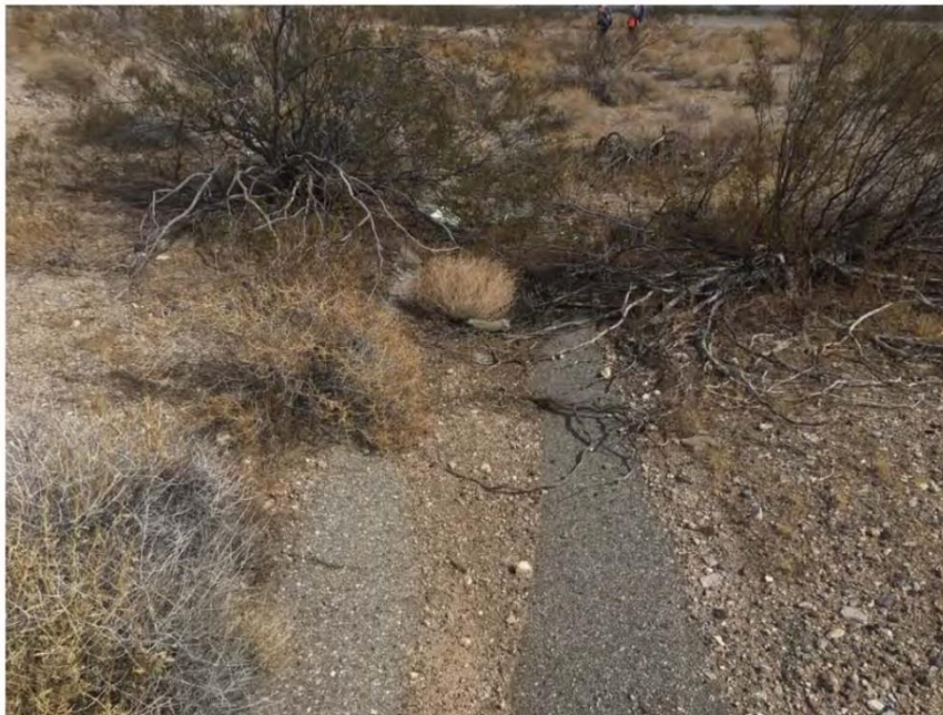
Photo 18: Non-jurisdictional concrete-lined v-ditch, facing east.
