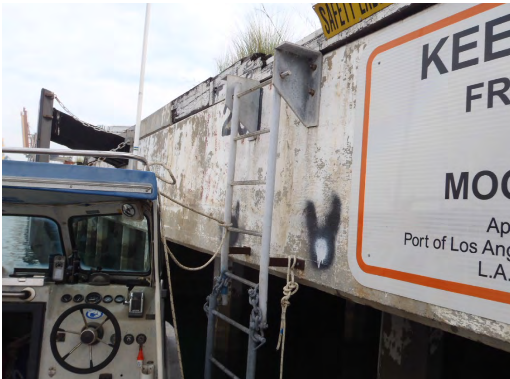
Photo 40: IA-01, retrieval line tied to ladder
