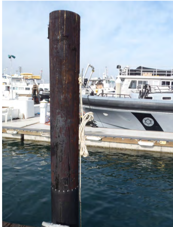
Photo 37: FH-01, retrieval line tied to cleat of the piling
