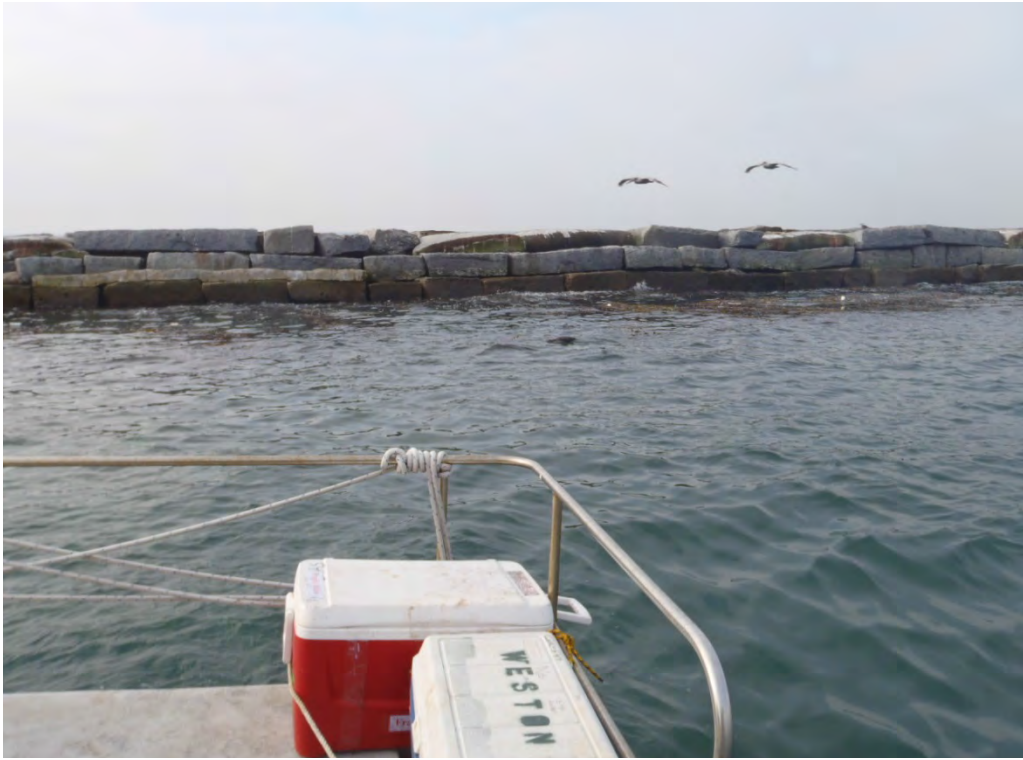
Photo 31: CP-01, facing southwest
