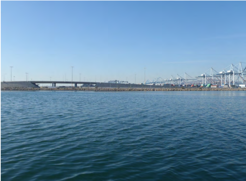
Photo 13: OB-01, facing west
