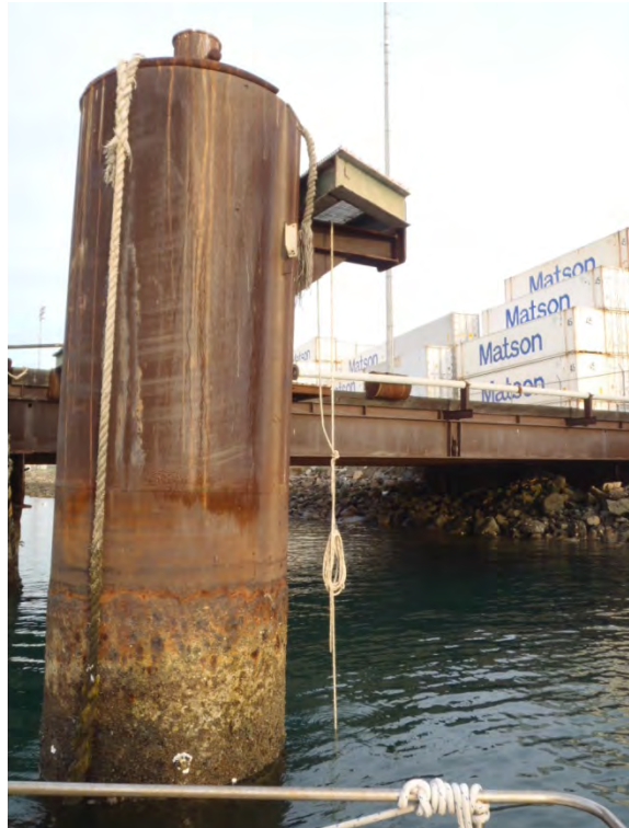
Photo 47: IB-01, facing northeast, retrieval line tied to overhead beam on piling
