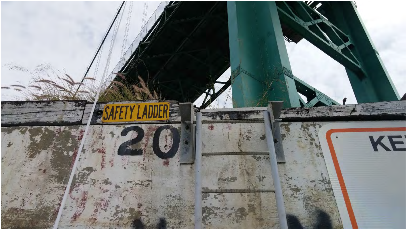
Photo 13: Signage at IA-01 location
