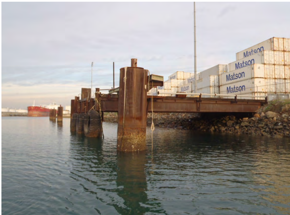
Photo 48: IB-01, facing northeast, retrieval line tied to overhead beam on piling
