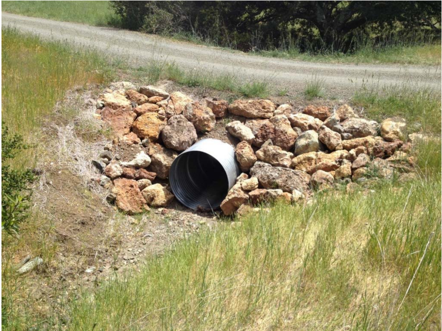
PWA Site #5 inlet (May 2014)
