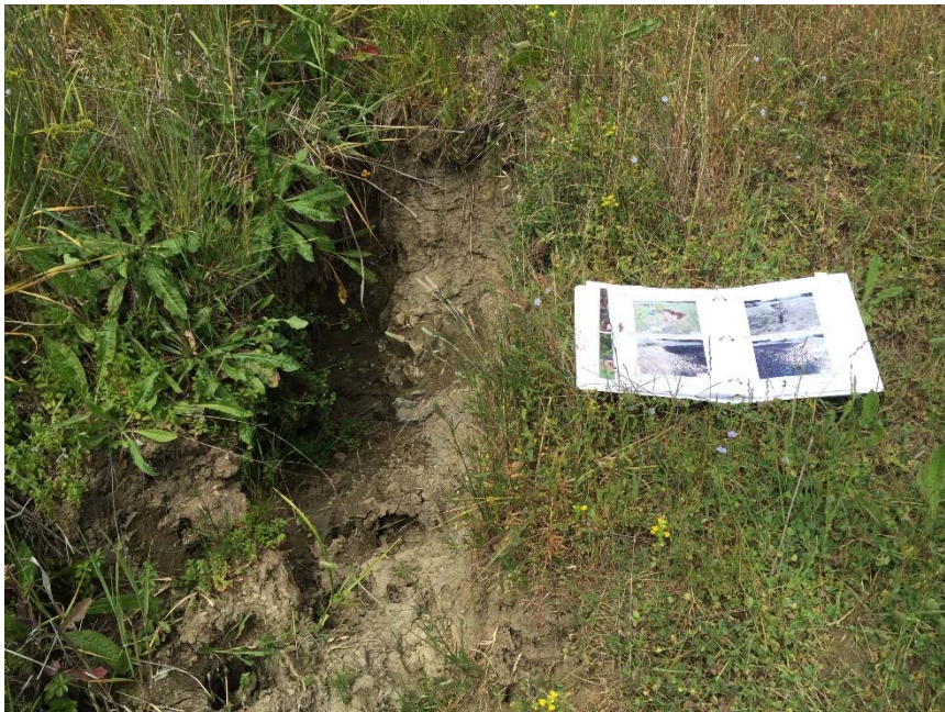
Additional view of headcut above PWA Site #6.2, below PWA Site #8.1 (May 2015)
