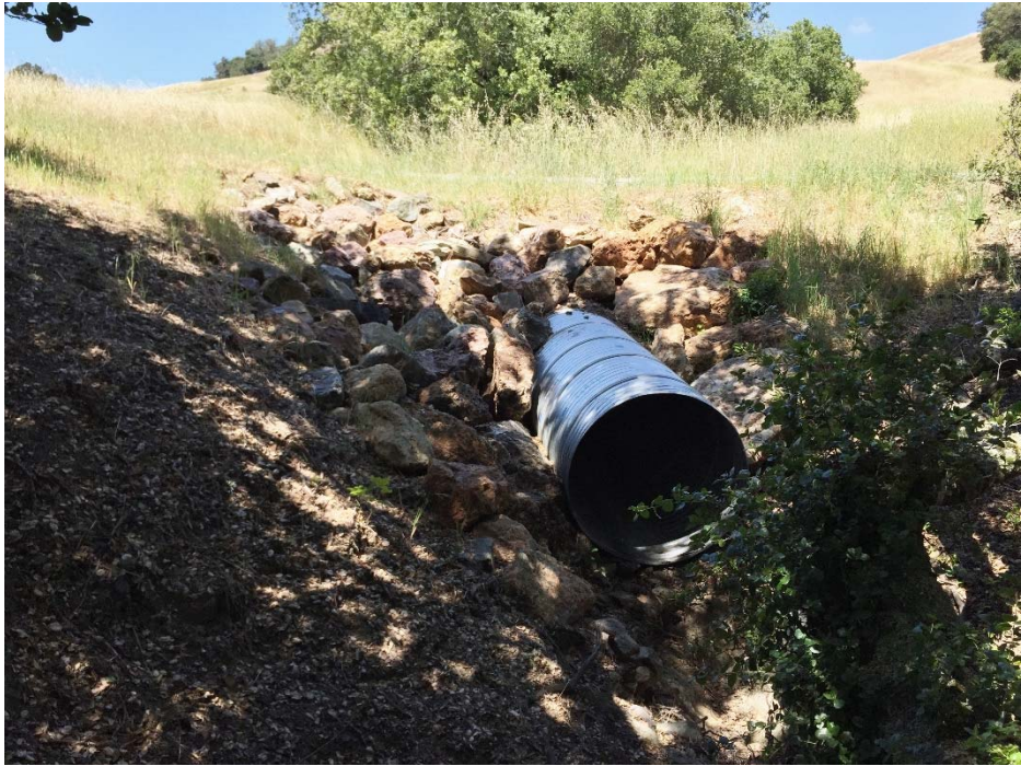
PWA Site #5 outlet (May 2015)
