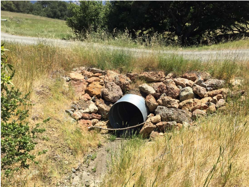
PWA Site #5 inlet (May 2015)
