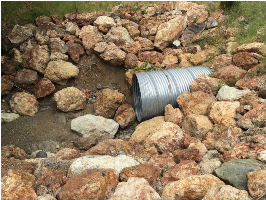
PWA Site #6 outlet (May 2015)
