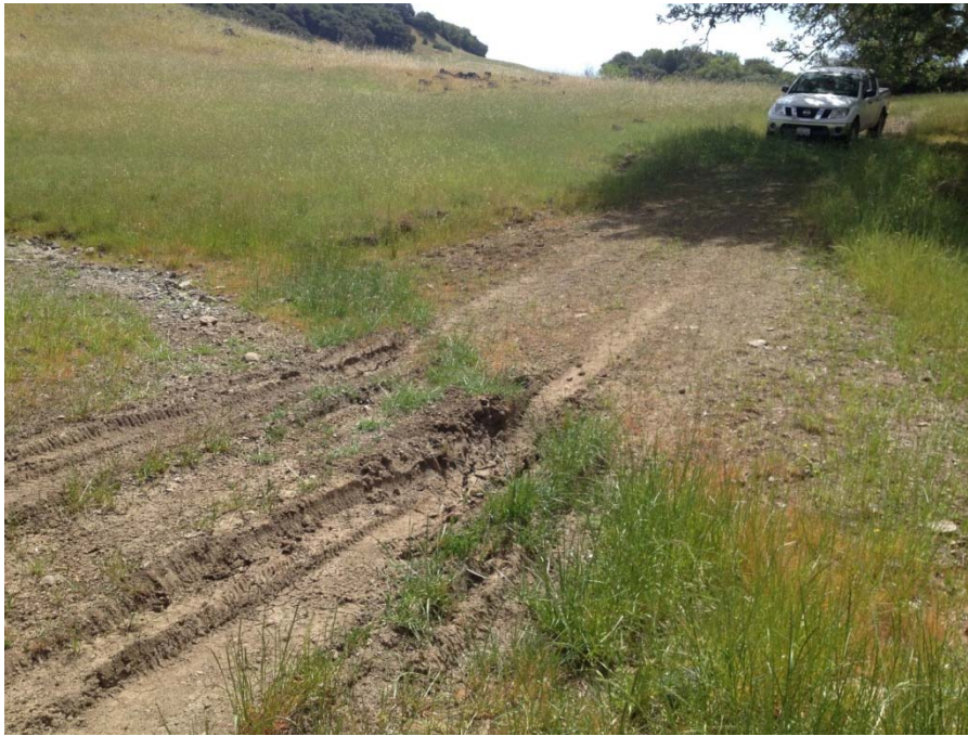
PWA Site # 33 – Tire ruts in road (May 2014)
