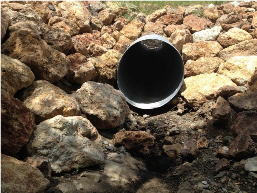
PWA Site #6 outlet (May 2014)
