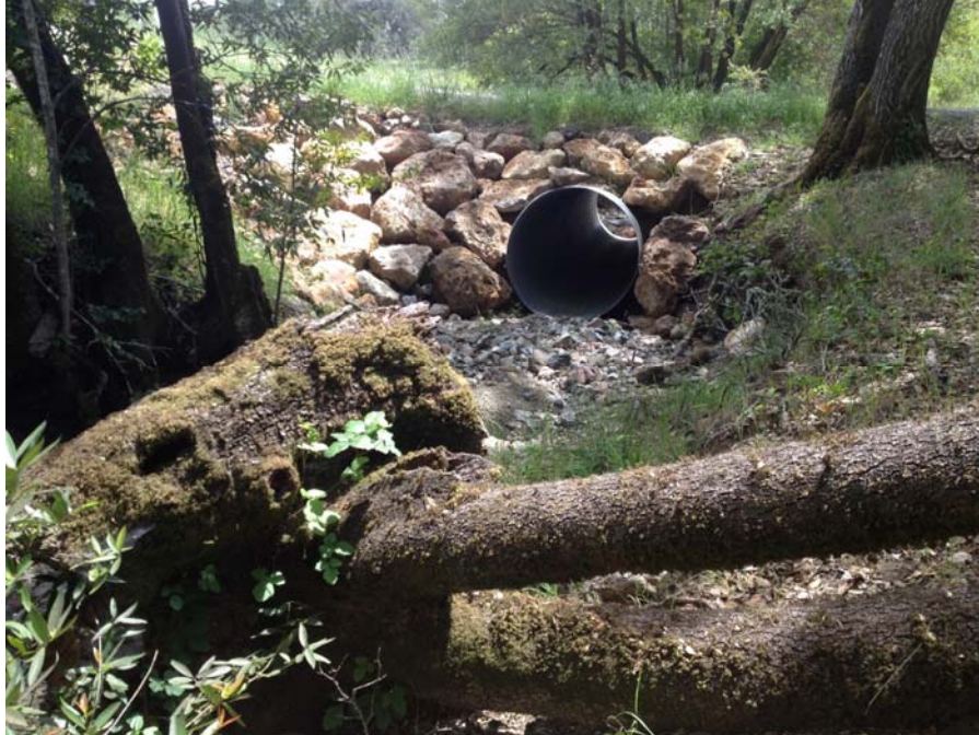
PWA Site #6 inlet (May 2014)
