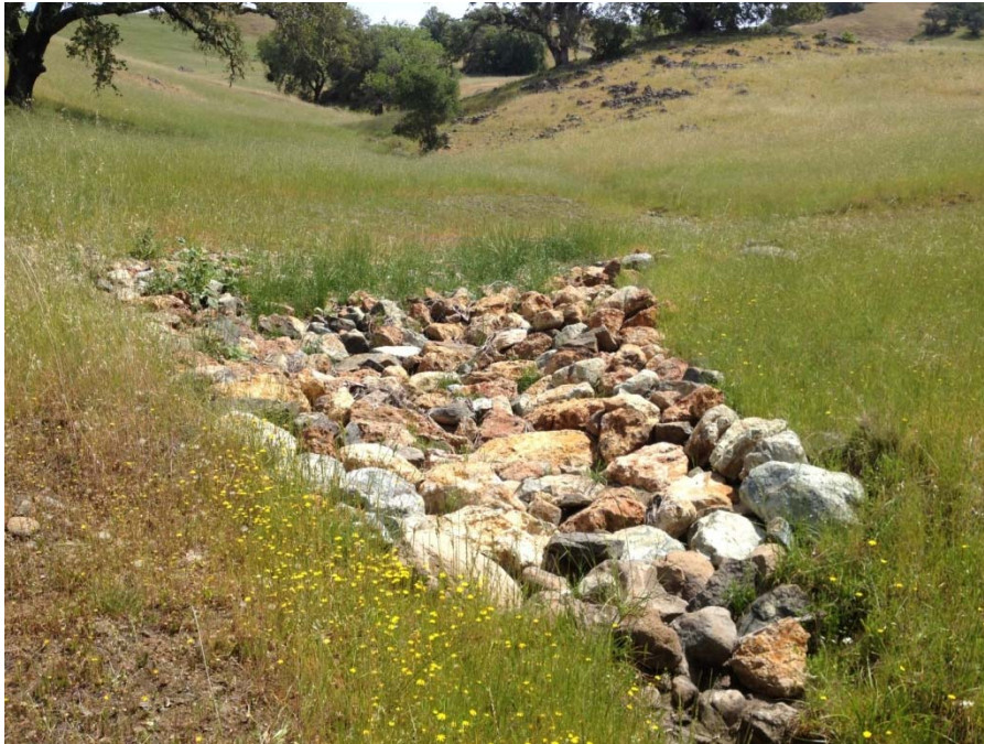
PWA Site #33 uphill (May 2014)
