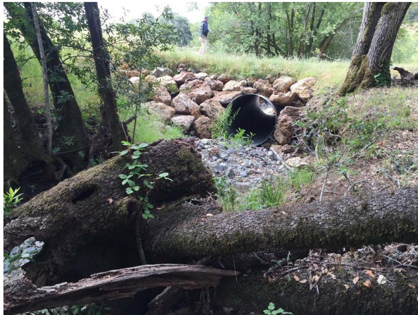
PWA Site #6 inlet (May 2015)
