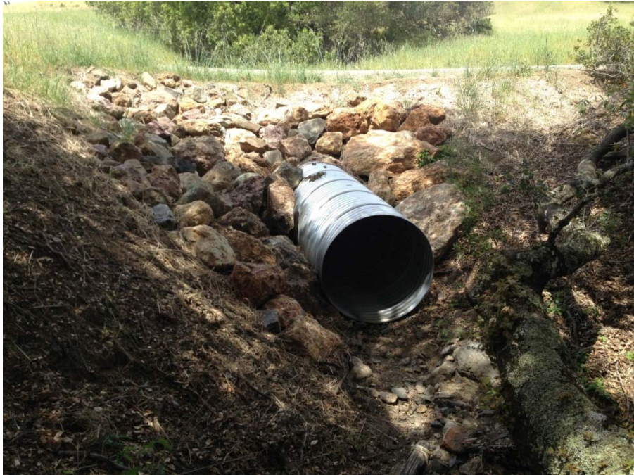
PWA Site #5 outlet (May 2014)
