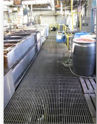
Metal plating shop. Credit: Los Angeles Regional Water Board
