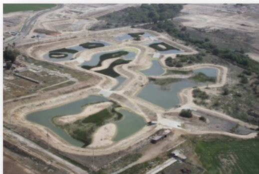
Millcreek Wetlands. Credit: City of Ontario
