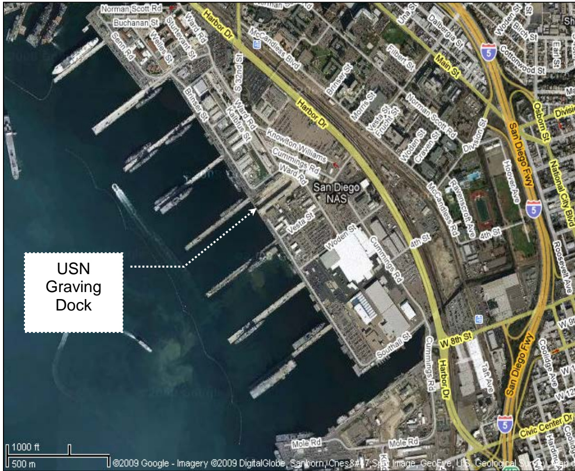
Figure B-9. USN Graving Dock at NBSD
