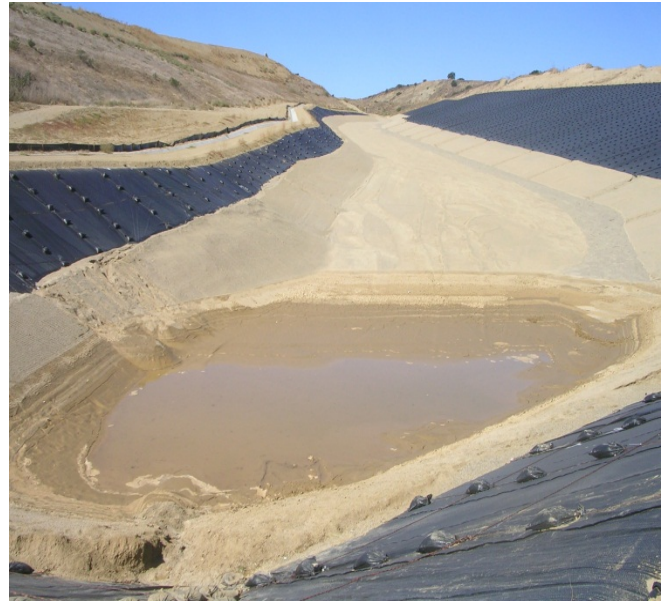
Damage to protective cover soils and ponding of storm water in Phase II expansion unit, Las Pulgas Landfill
