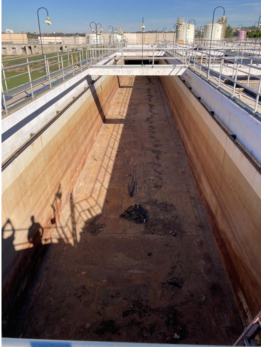
Figure 5: PST 5 Under Repair (DWG 11-22-23).
