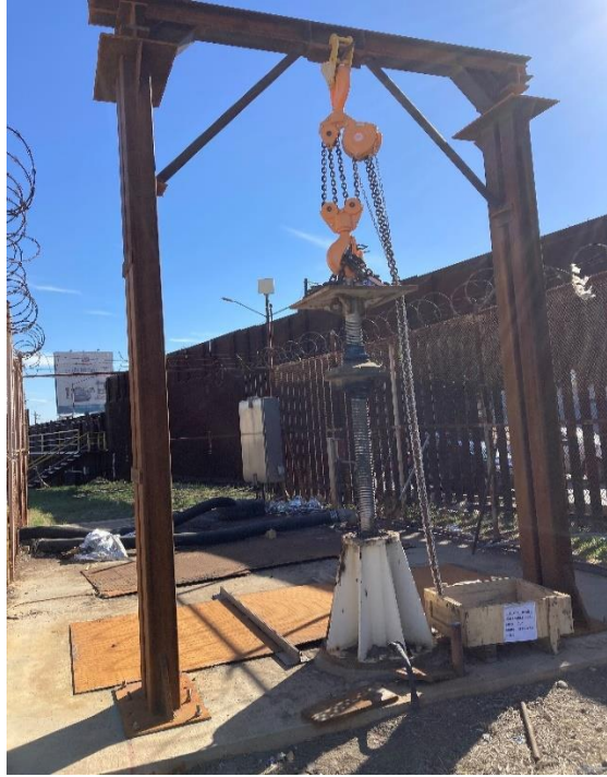
Figure 1: JB1 Interim Repairs in place (DWG 11-22-23).
