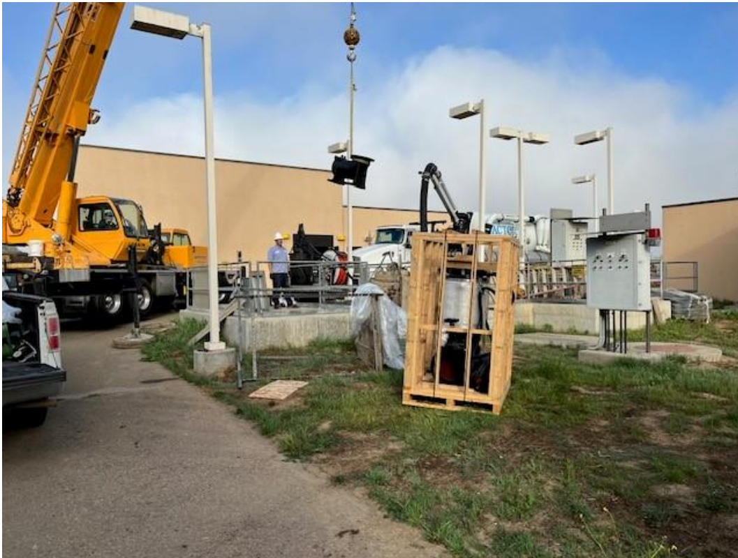
Figure 7: New pump being delivered to Hollister Ave. Pump Station (IBWC 10-16-23)
