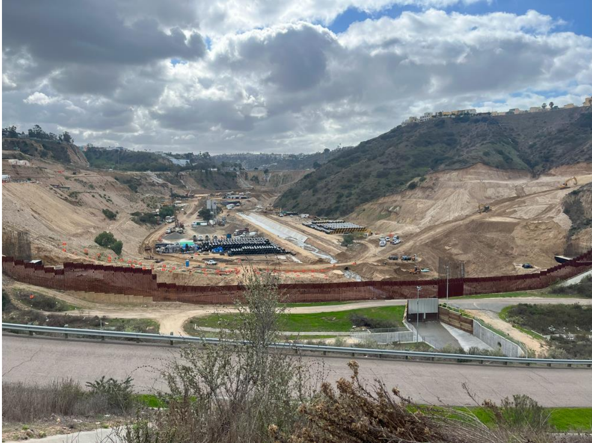
Figure 10: Mexican construction project in Matadero Canyon. (MC 01/10/2024)
