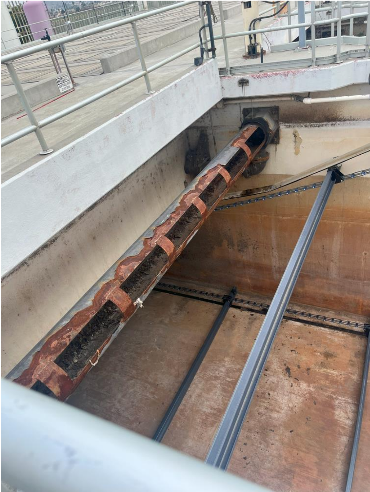
Figure 6: Existing skimmer trough at PST No. 5. (MC 01/10/2024)
