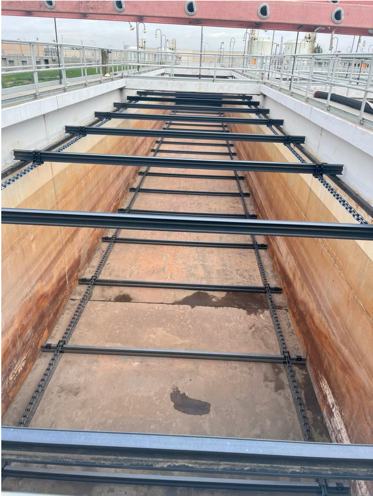
Figure 5: PST No. 5, rehabilitation complete. (MC 01/10/2024)
