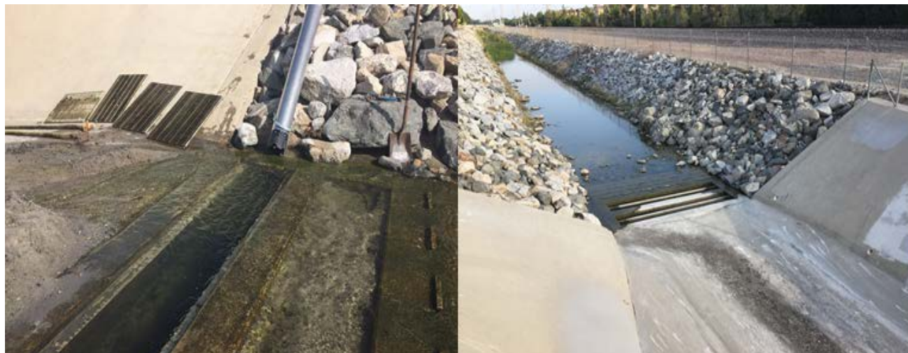
Figure 8: Peters Canyon Channel Water Capture and Reuse Diversion Project
