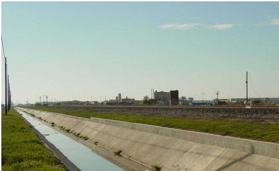
Figure 6: Revolon Slough, subject to the Revolon Slough/Beardsley Wash Trash TMDL
