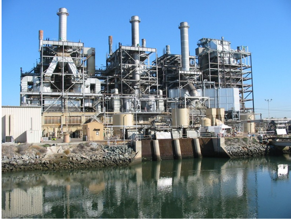
Figure 3-2. South Bay Power Plant showing the intake screenhouse for Units 1& 2.
