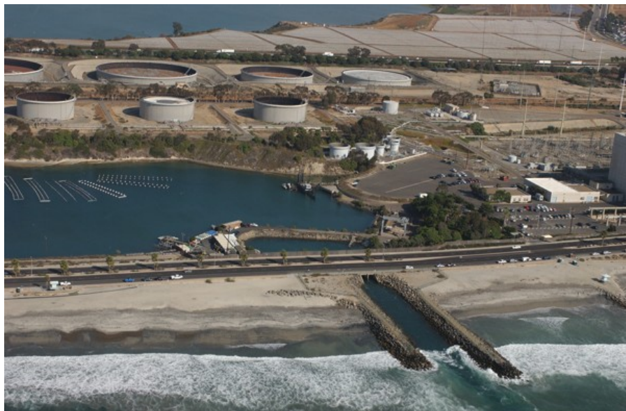
Figure 3-4. Encina Power Station cooling system intake and shoreline discharge.
