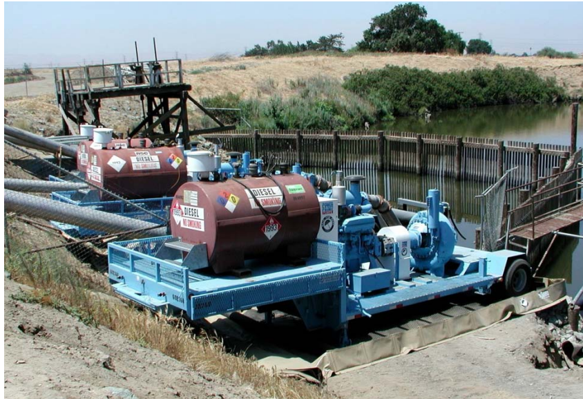
Figure III.9: Example of Temporary Pump and Generator Units
