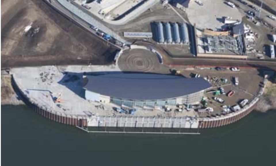
Figure 1: Example of an On-Bank Intake – FRWA Intake on the Sacramento River
