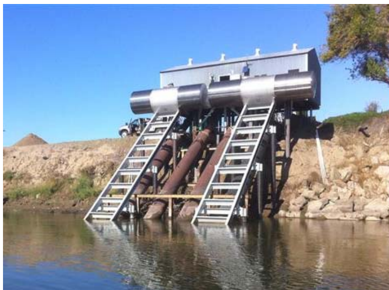
Figure III.8: Example of Cylindrical Screen Intake – SMWC State Ranch PP Temporary Cylindrical Screen Intakes
