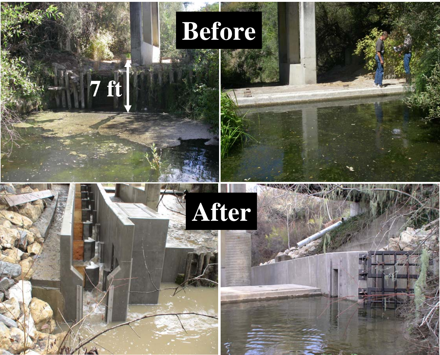
Figure 10: Fish passage and habitat restoration in the fall of 2008 at Rancho San Julian on El Jaro Creek.
