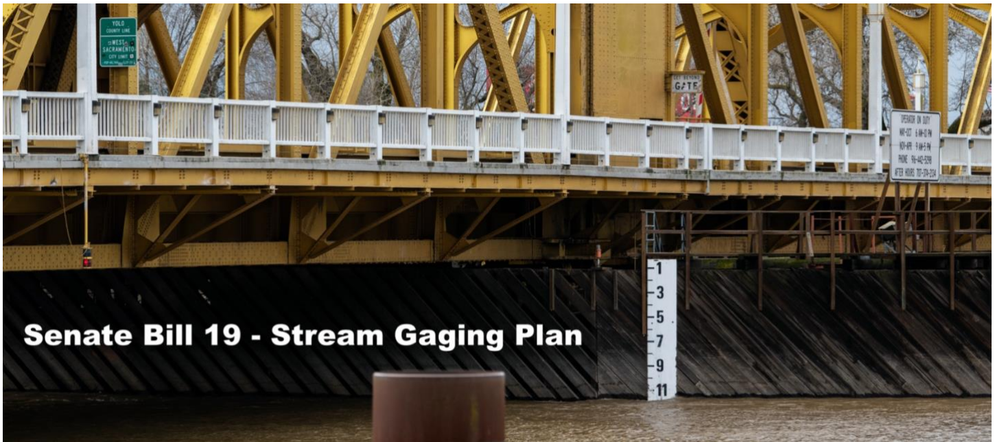
Figure 1. A river gauge marker located beside the Tower Bridge in Sacramento, California, measures the water level on the Sacramento River.
